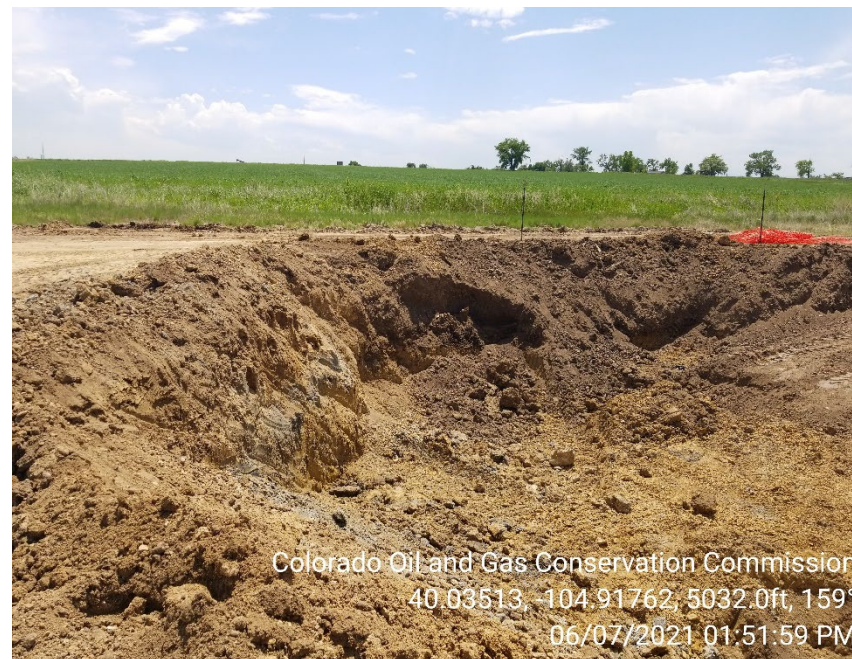
Photo 4 – Open excavation. Impacts remain in situ. Excavation appears to have been partially backfilled.
