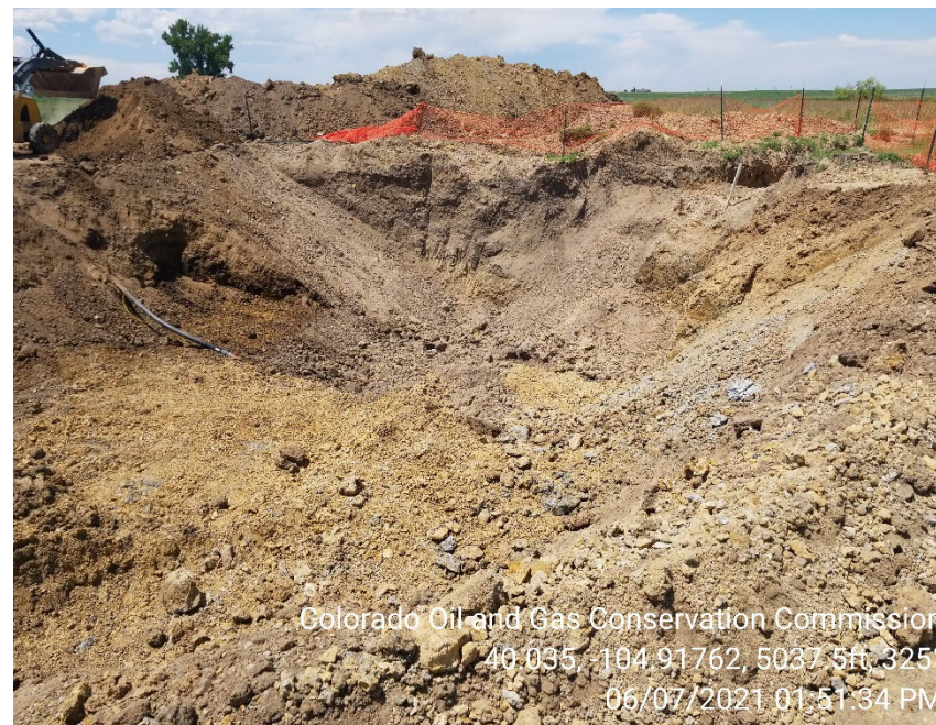
Photo 2 – Open excavation. Excavation appears to have been partially backfilled.
