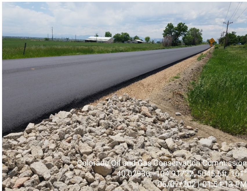
Photo 5 – Vehicle tracking BMPs have been installed and dirt previously carried of location has been removed/cleaned.
