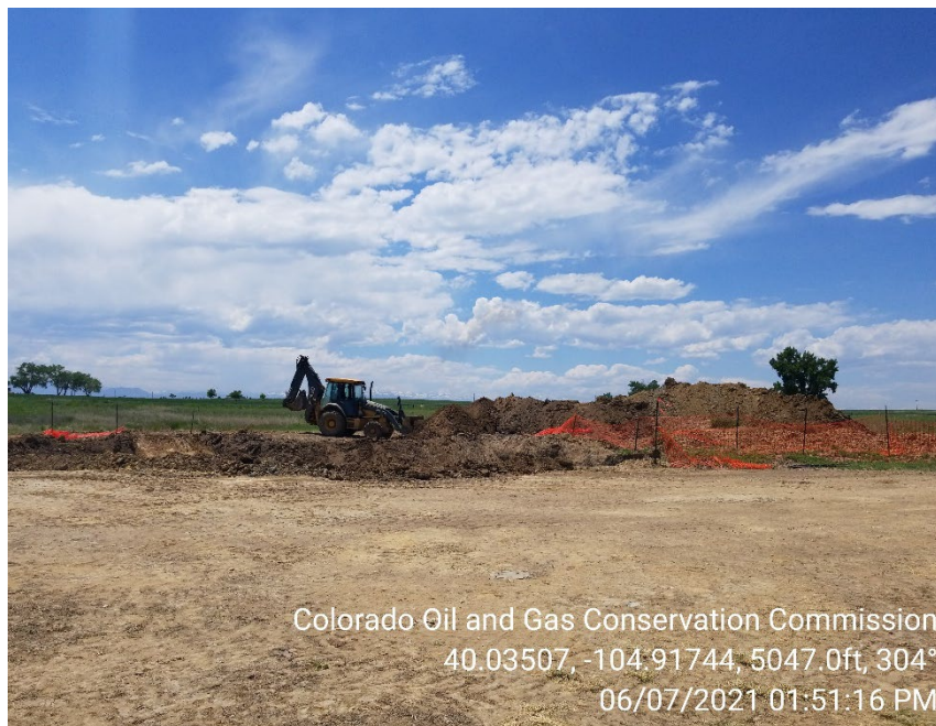
Photo 1 – Spill area. Excavation in process at the time of the inspection.
