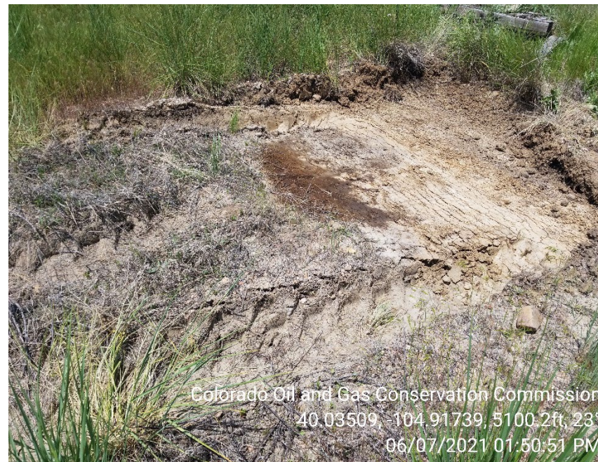
Photo 6 – New Spill (spill ID 480128). Surface area has been scraped. Impacts remain in situ and visible on the surface.
