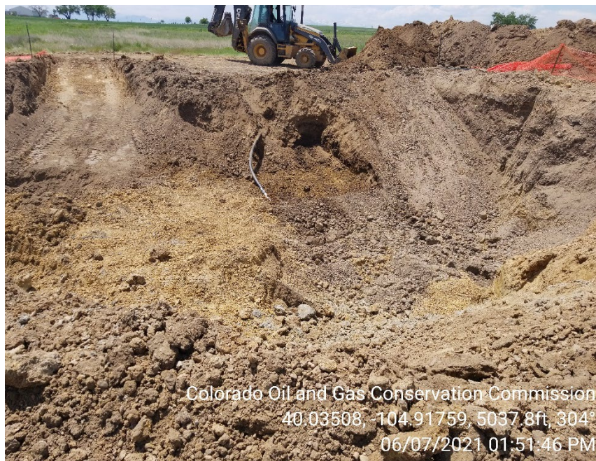
Photo 3 – Open excavation. Area where free product was previously observed appears to have been partially backfilled.
