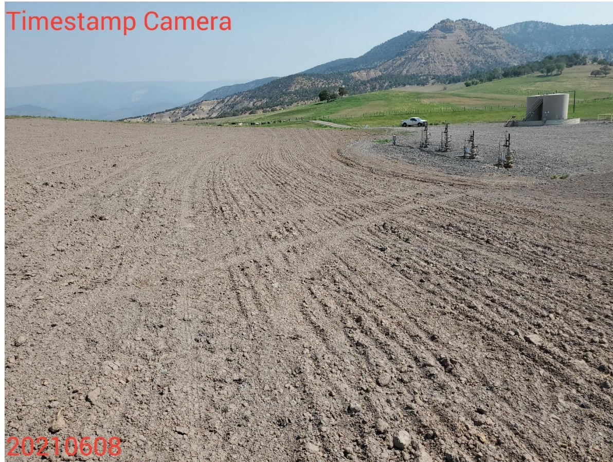
Photo 4: Photo taken from the southwestern area of the location, facing north. Photo shows additional reclamation and revegetation activities have been conducted. Photo also shows control measures to stabilize the soils and slopes of the Location are missing or insufficient.
