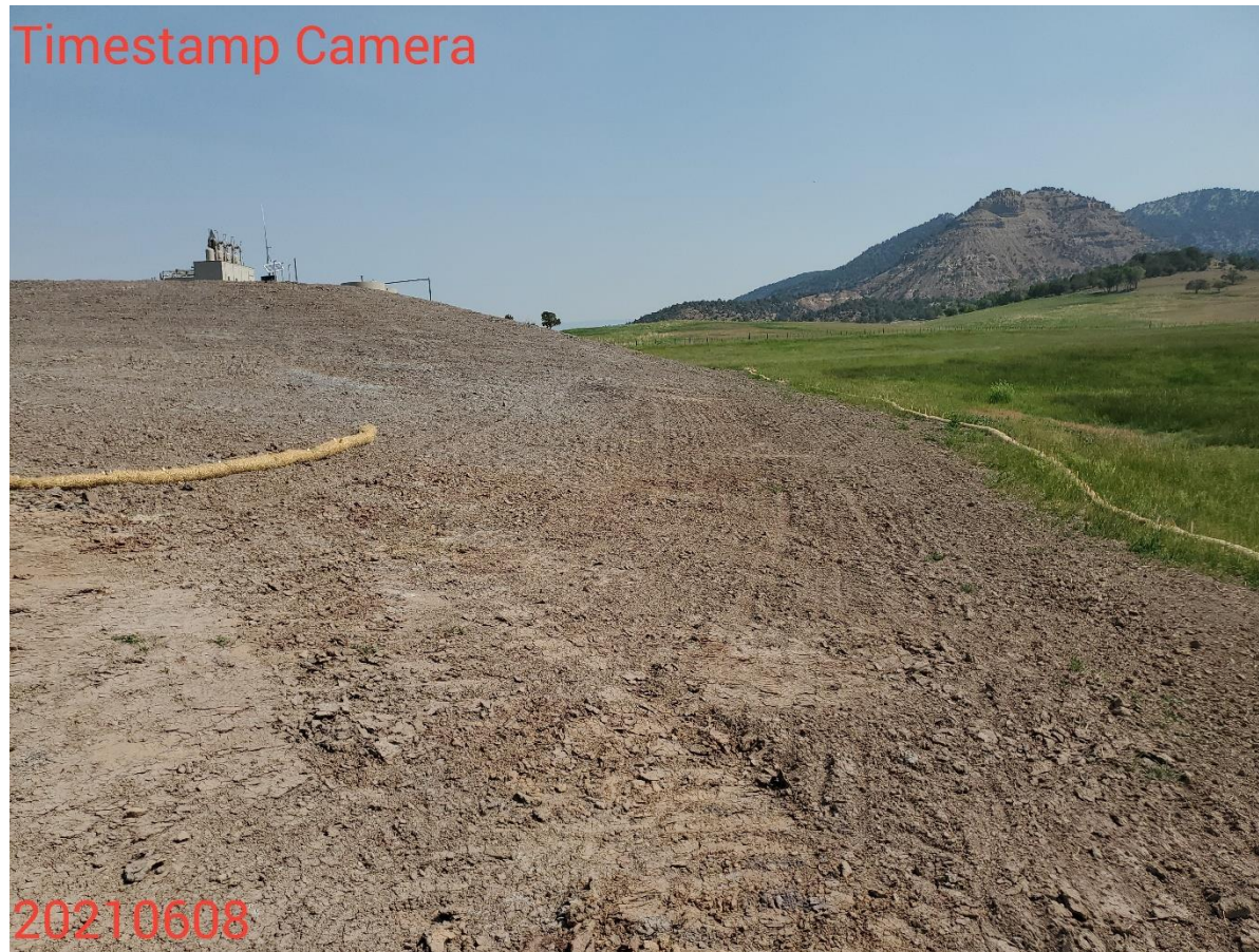
Photo 7: Photo taken from the southeastern area of the location, facing north. Photo shows additional reclamation and revegetation activities have been conducted. Photo also shows control measures to stabilize the soils and slopes of the Location are missing or insufficient.
