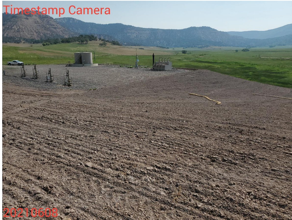
Photo 5: Photo taken from the southwestern area of the location, facing northeast. Photo shows additional reclamation and revegetation activities have been conducted. Photo also shows control measures to stabilize the soils and slopes of the Location are missing or insufficient.
