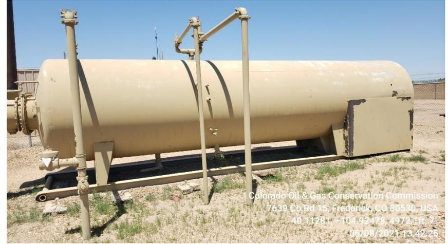
**Photo 7 Horizontal Heated Separator**
