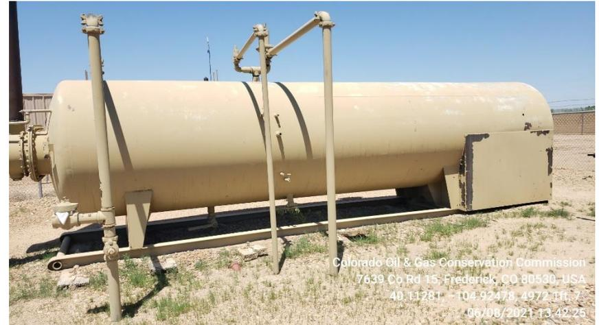
**Photo 7 Horizontal Heated Separator**
