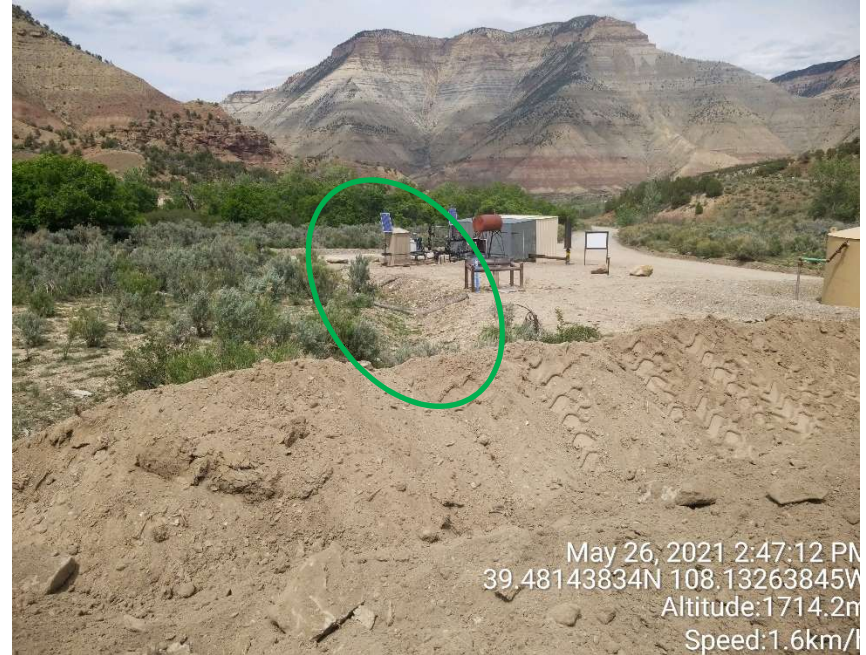
Land Treatment area built across an un-named, dry arroyo. Note where the un-named dry arroyo is visible on the northern end of the Land Treatment area (green oval).
