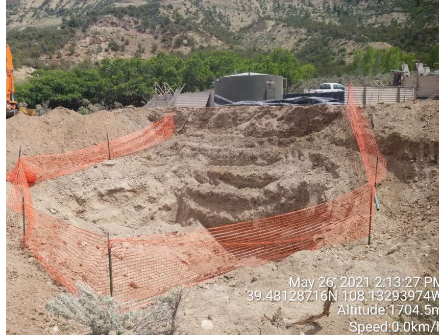
Excavation looking towards the tank battery where the spill/release originated. Note the tank battery secondary containment in disrepair.
