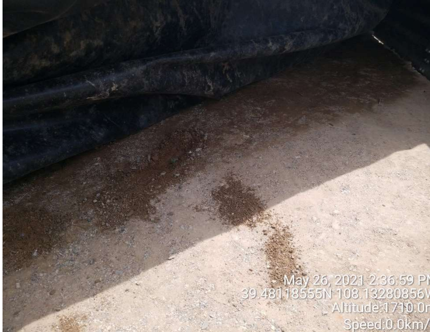
Potentially impacted material underneath the liner of the secondary containment structure around the northwest corner of the tank battery.
