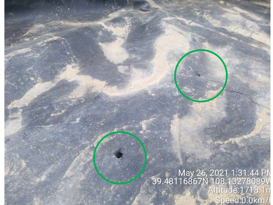
Additional holes in the liner of the secondary containment structure (green circles).
