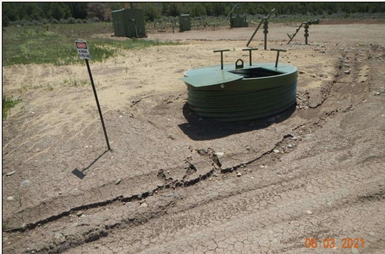
Photos 4. View of erosional rilling at well pad entrance. Stormwater BMPs need to be installed and maintained until area is stabilized with desirable perennial vegetation.
