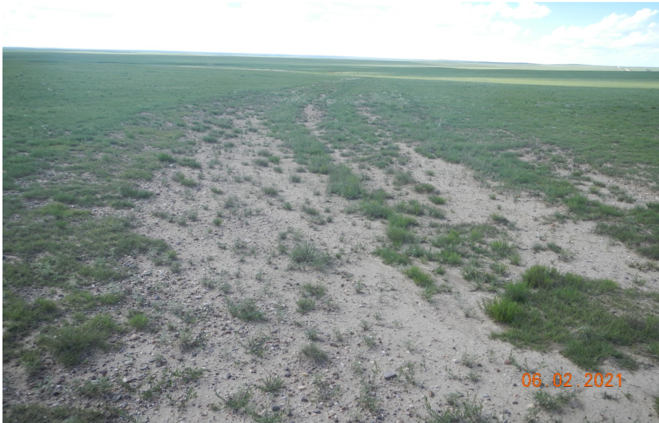
Photo 5. Facing northwest along the former access road. The majority of the road has re-established vegetation. The area where the road turns has bare areas that will needed addition reclamation.
