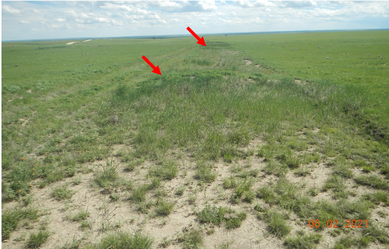
Photo 4. Facing south along the former access road. There are multiple berms along the former road that need to be leveled and reclaimed.
