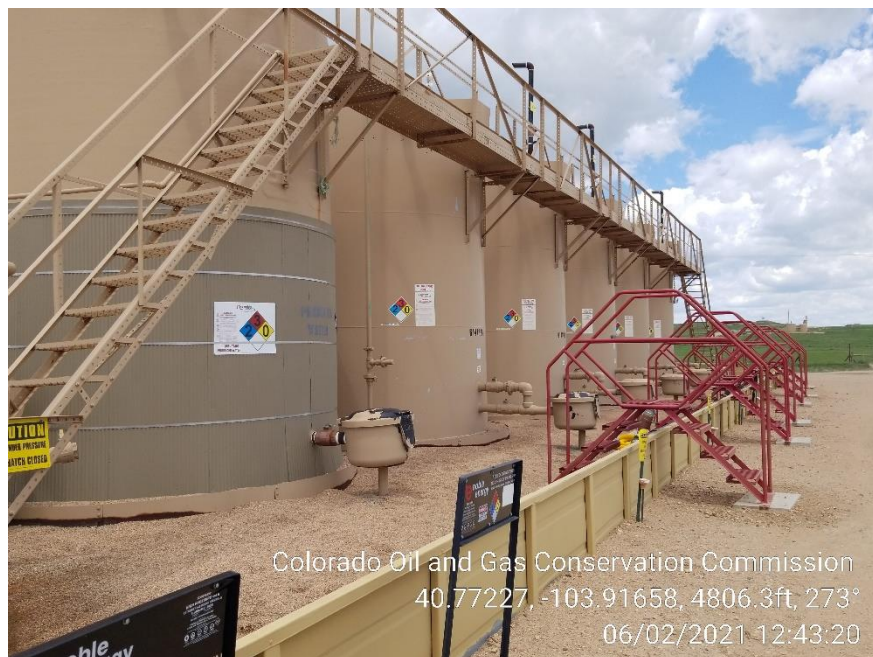
Photo 5 – Tank Battery
