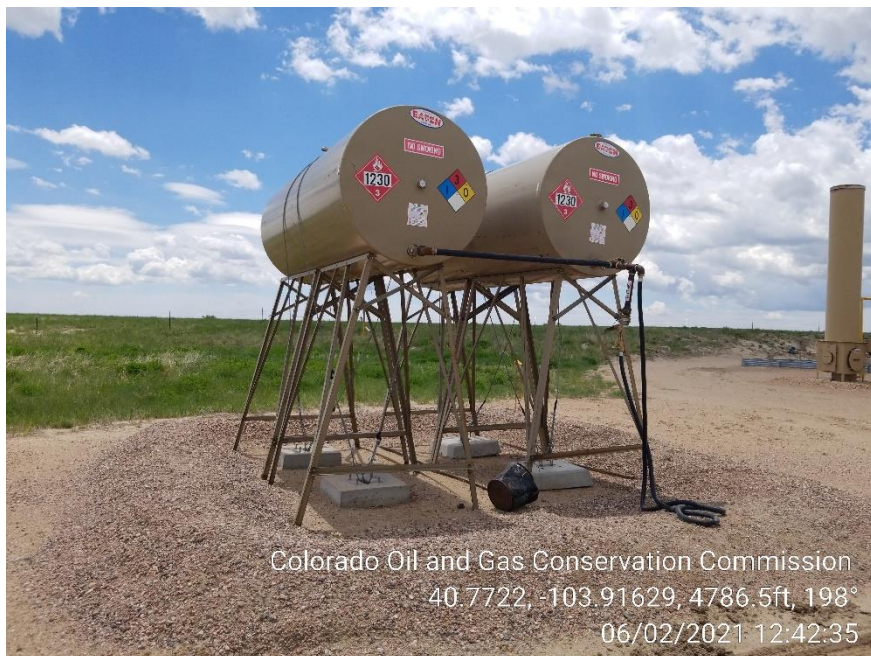
Photo 3 – Methanol Day Tanks
