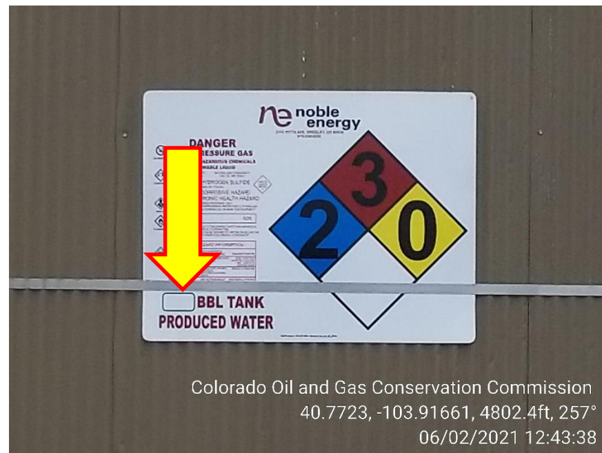
Photo 10 – Capacity Label Missing
