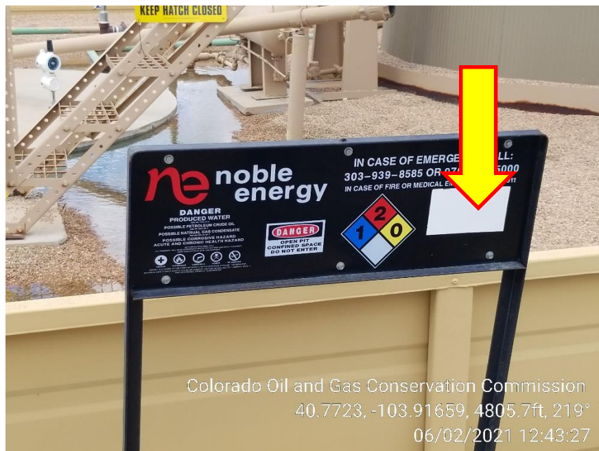
Photo 9 – Capacity Label Missing
