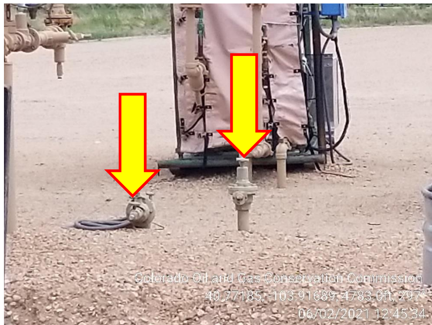
Photo 7 – Unmarked Risers at Compressor
