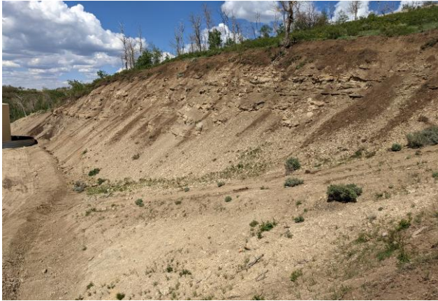
Containment Berm Installed below CC 610-22-43 Cut Slope
