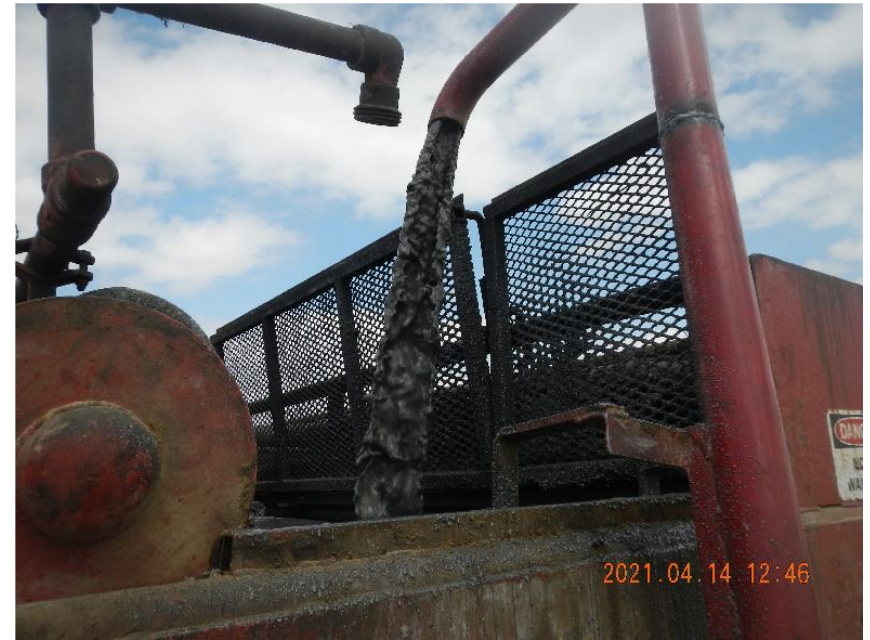
Photo 2: Returns to the surface during cement plug milling.
