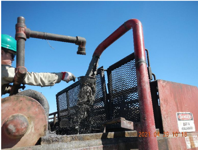
Photo 7: View of returns to surface as wash down work continues.
