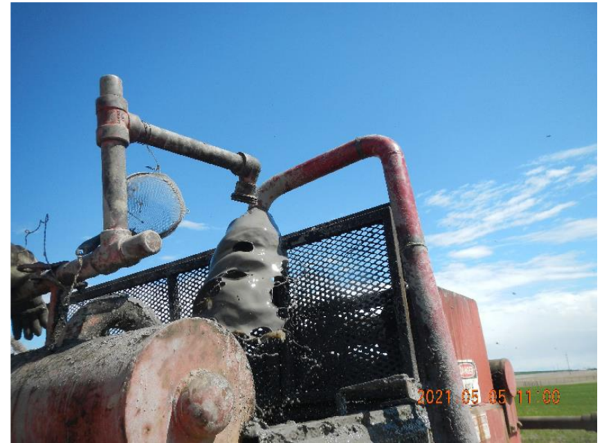
Photo 12: Good returns to the surface while pumping cement.
