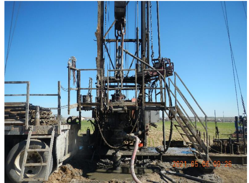
Photo 14: Cementing equipment rigged into well to pump surface casing plug.
