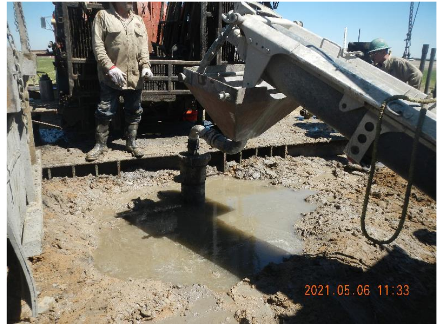
Photo 16: Topping off surface casing after rig down completed.
