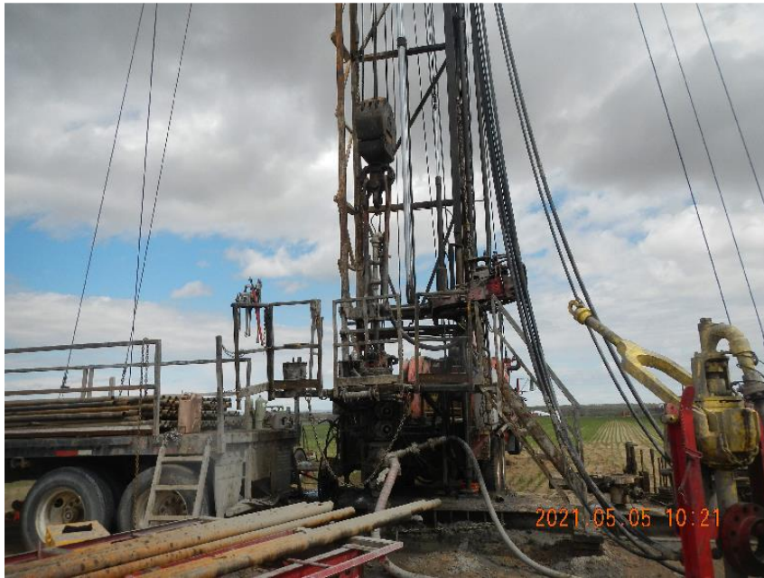
Photo 11: View of cementing equipment rigged into well to pump cement plug #2.
