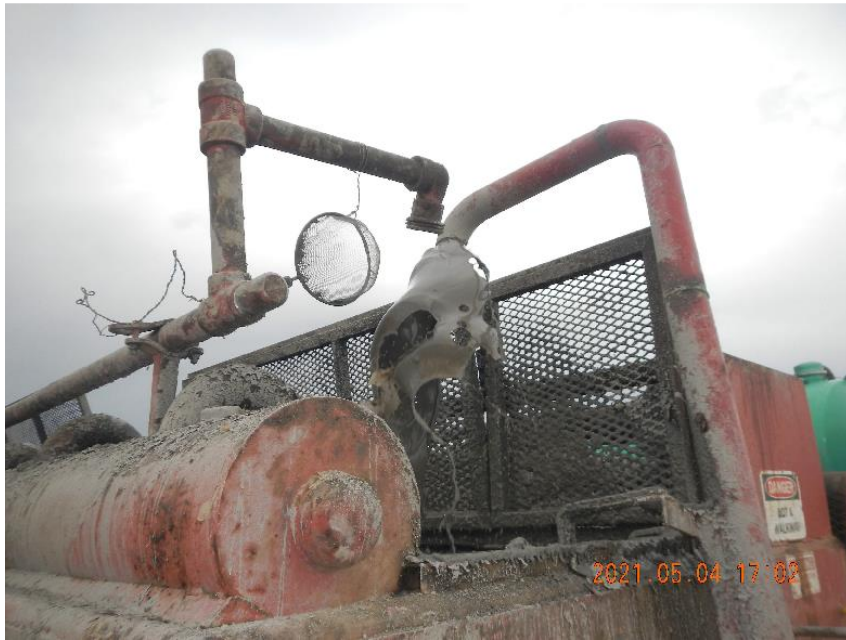
Photo 9: View of returns to the surface while pumping cement plug.
