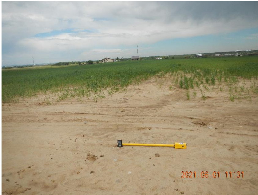
Photo 17: View of locator and Trimble GPS over surface casing after casing cut and capped.
