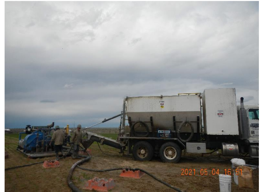
Photo 8: Crew preparing to pump new cement plug after reaching plug depth.
