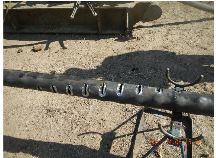
Photo 8: View of perforation tool after use. Casing perforated and ready for cement plug.
