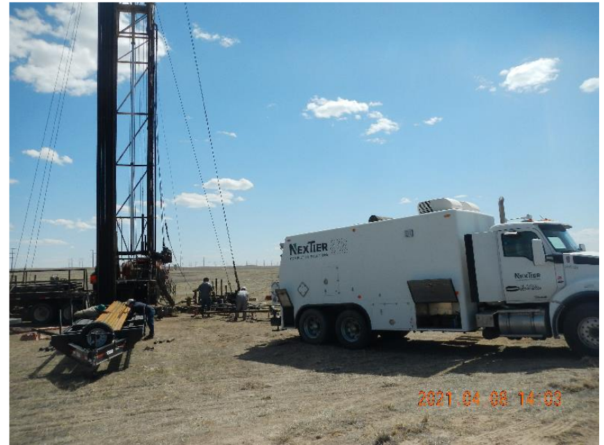
Photo 6: Wireline rigged into well to set cast iron bridge plug.
