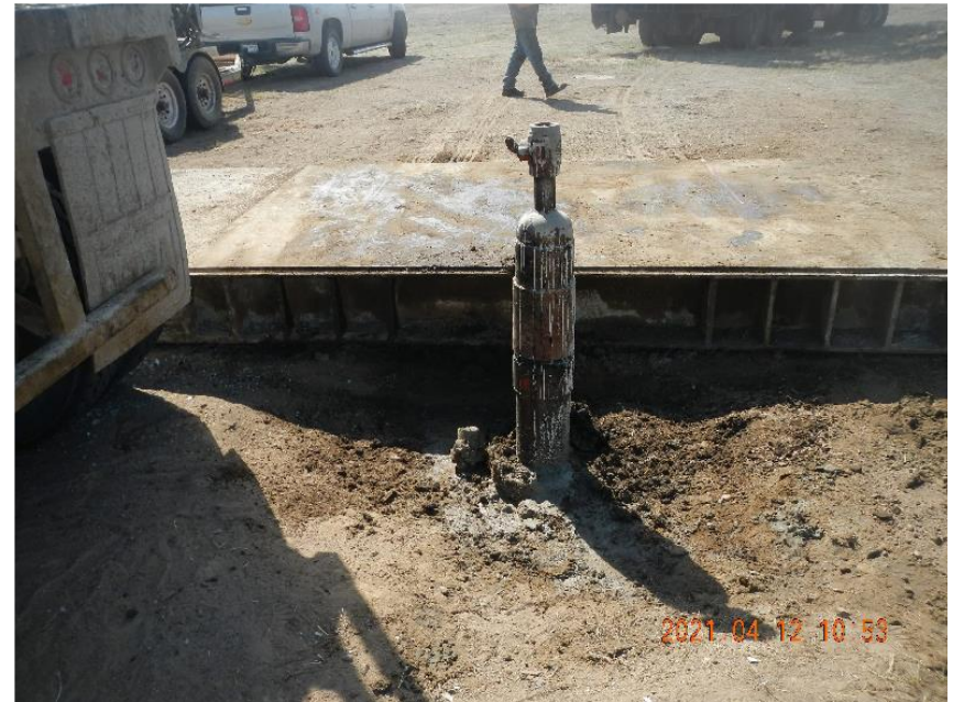
Photo 12: View of surface casing after plugging work completed. Surface casing will be cut and capped after 5 day wait period.
