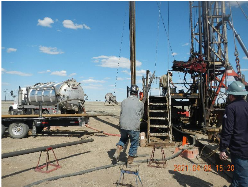
Photo 7: View of crew lifting perforation tool to go down hole for perforating casing for cement plug.
