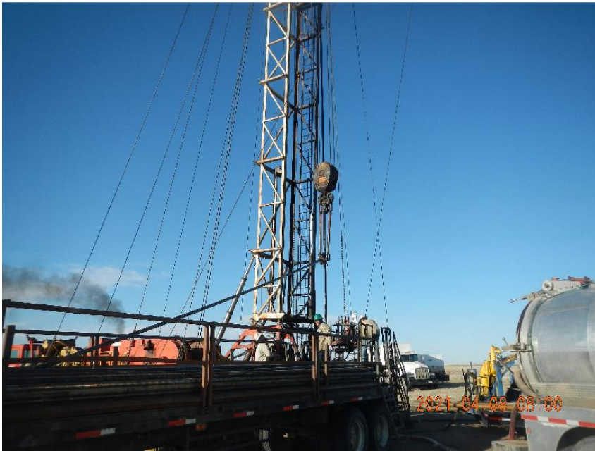
Photo 5: View of operations as crew trips work string into well.
