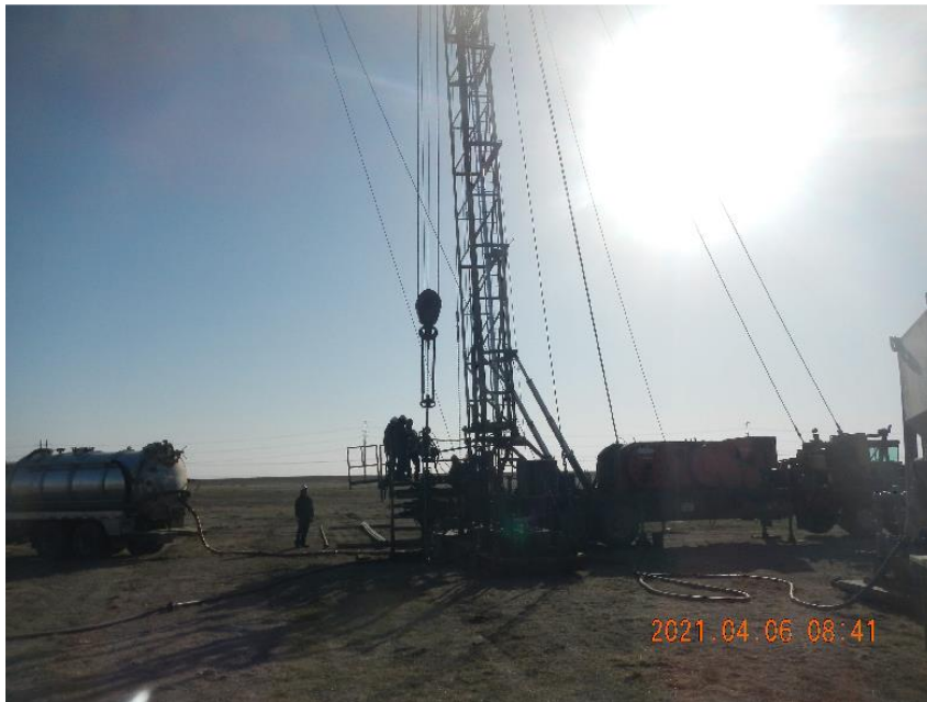
Photo 3: View of rig on well and crew tripping work string into well.
