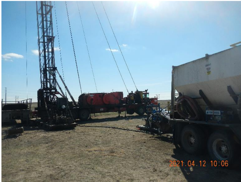
Photo 9: View of cementing equipment rigged in for cement work.
