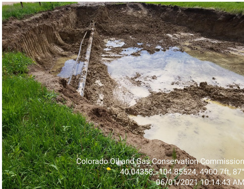
Photo 3 – Spill excavation. Hydrocarbons observed on groundwater in open excavation.
