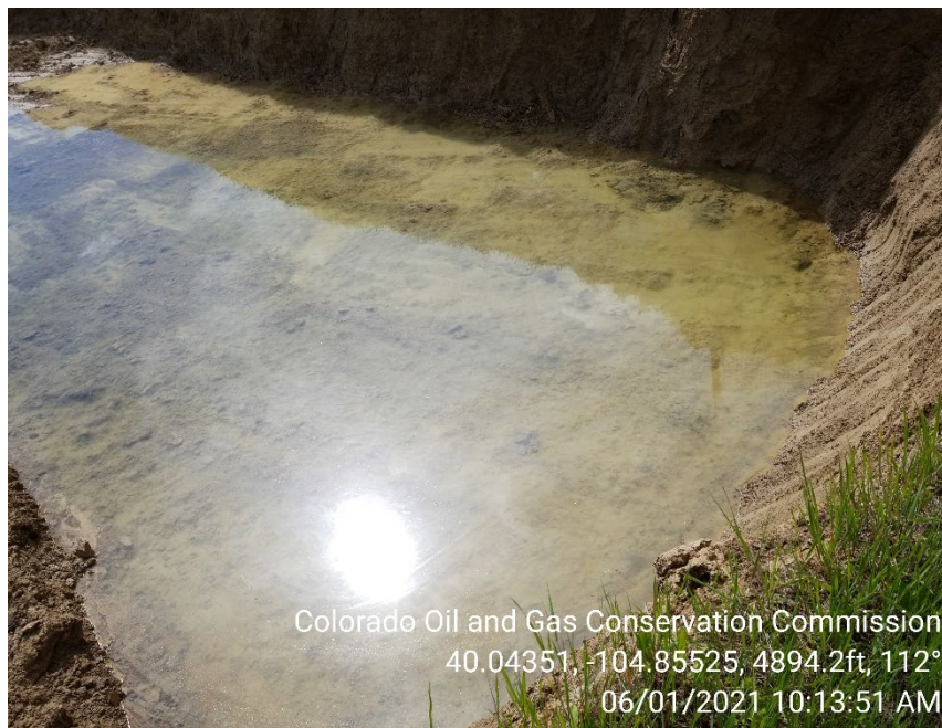
Photo 5 – Spill excavation. Hydrocarbons sheen observed on groundwater in open excavation.
