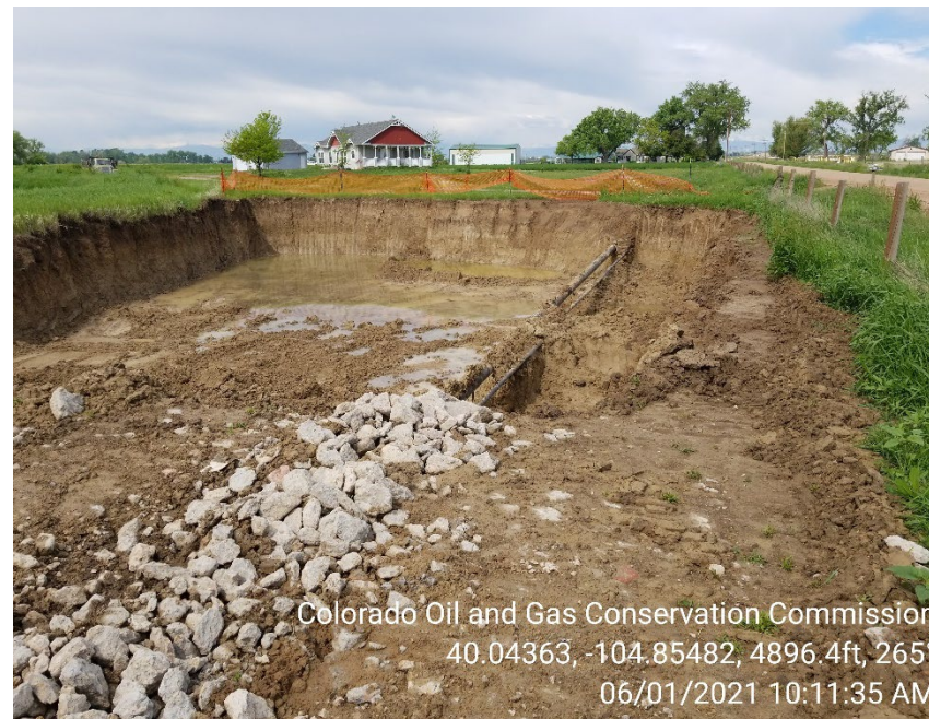
Photo 4 – Exposed flowline in open excavation.
