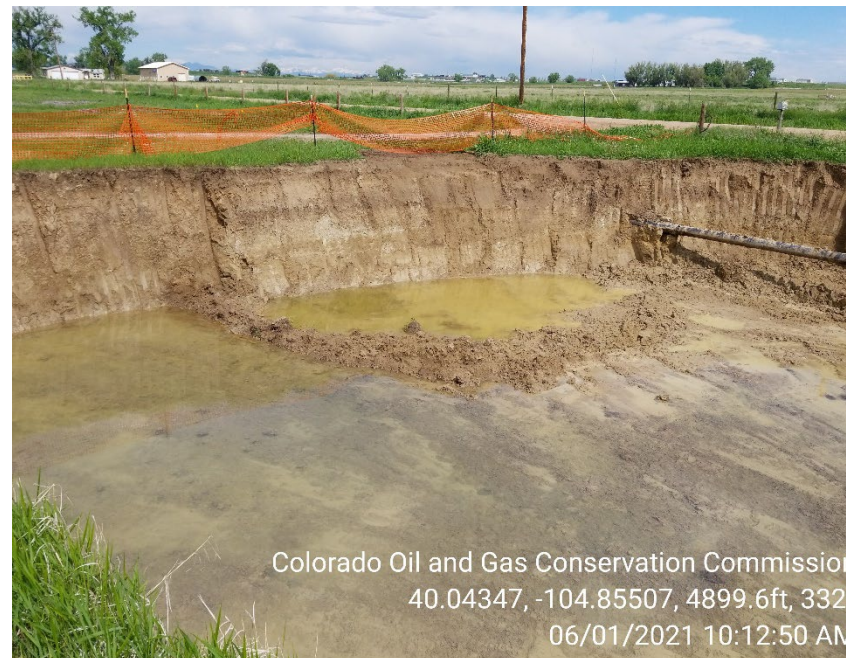
Photo 2 – Spill excavation. Groundwater with hydrocarbon sheen observed in open excavation.
