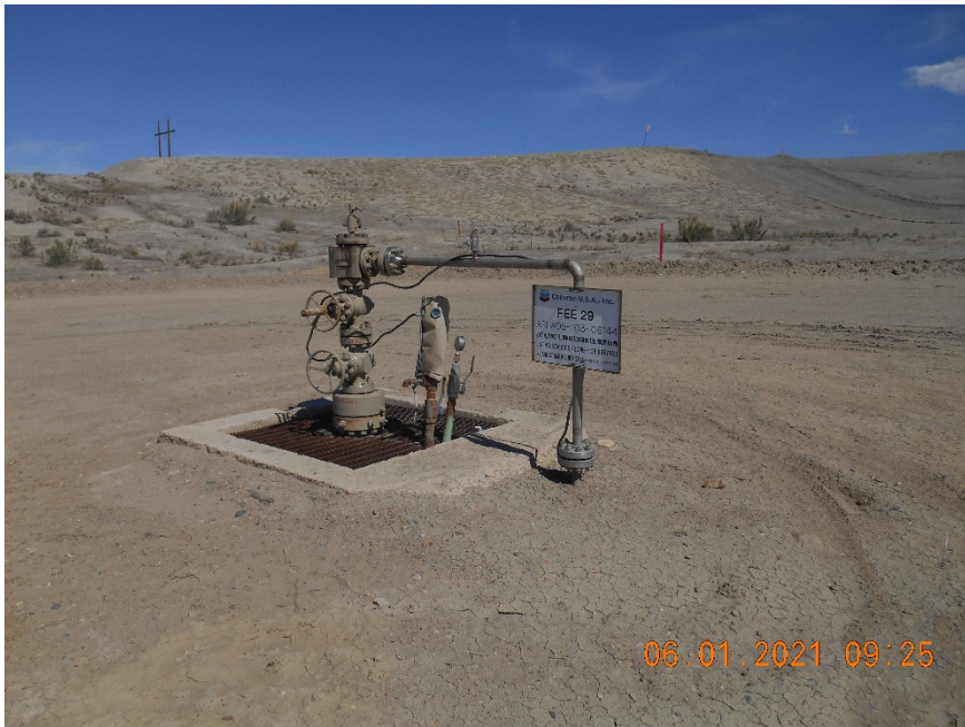
Injection wellhead.
