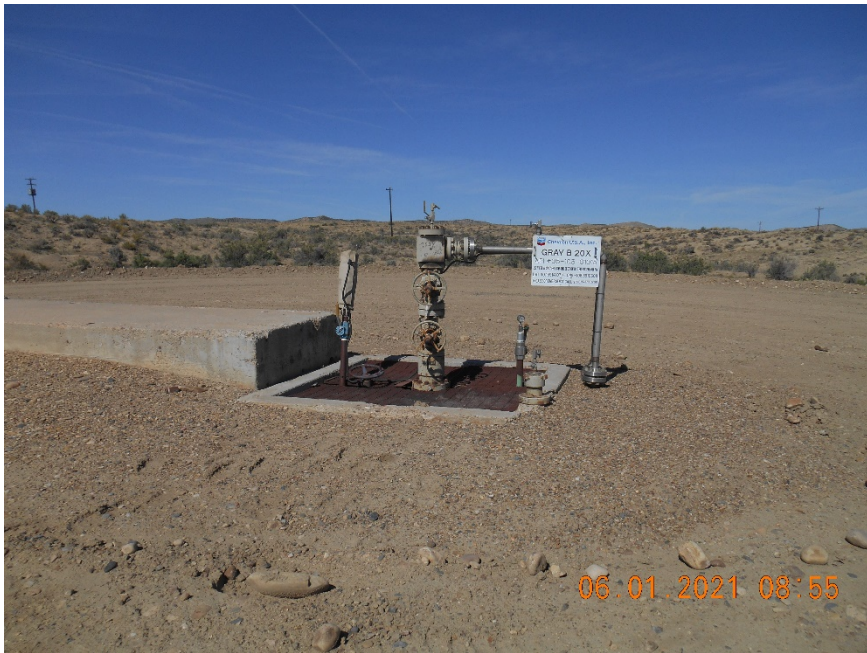
Injection wellhead
