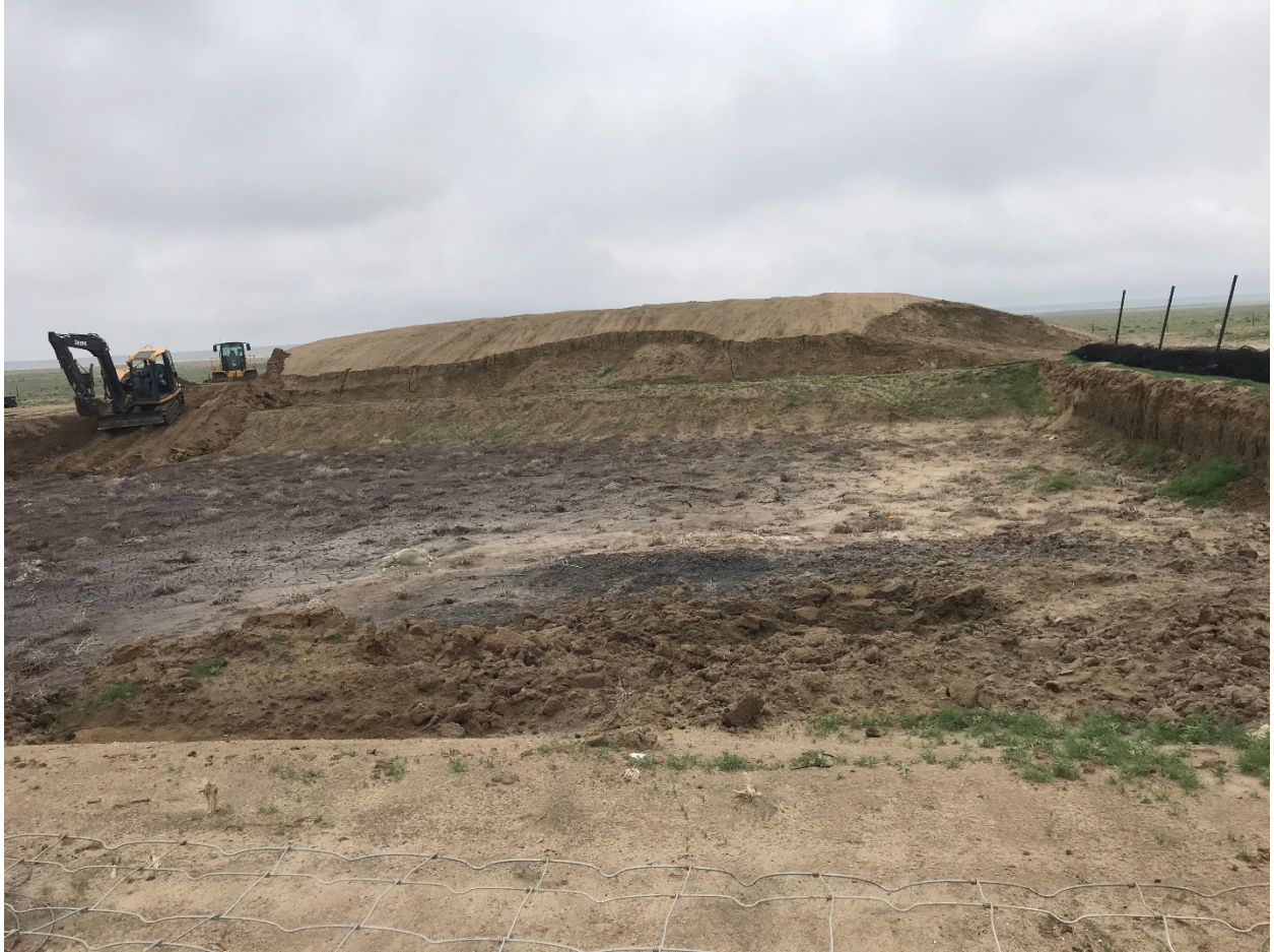
Pit prior to mixing facing west 5/15/21
