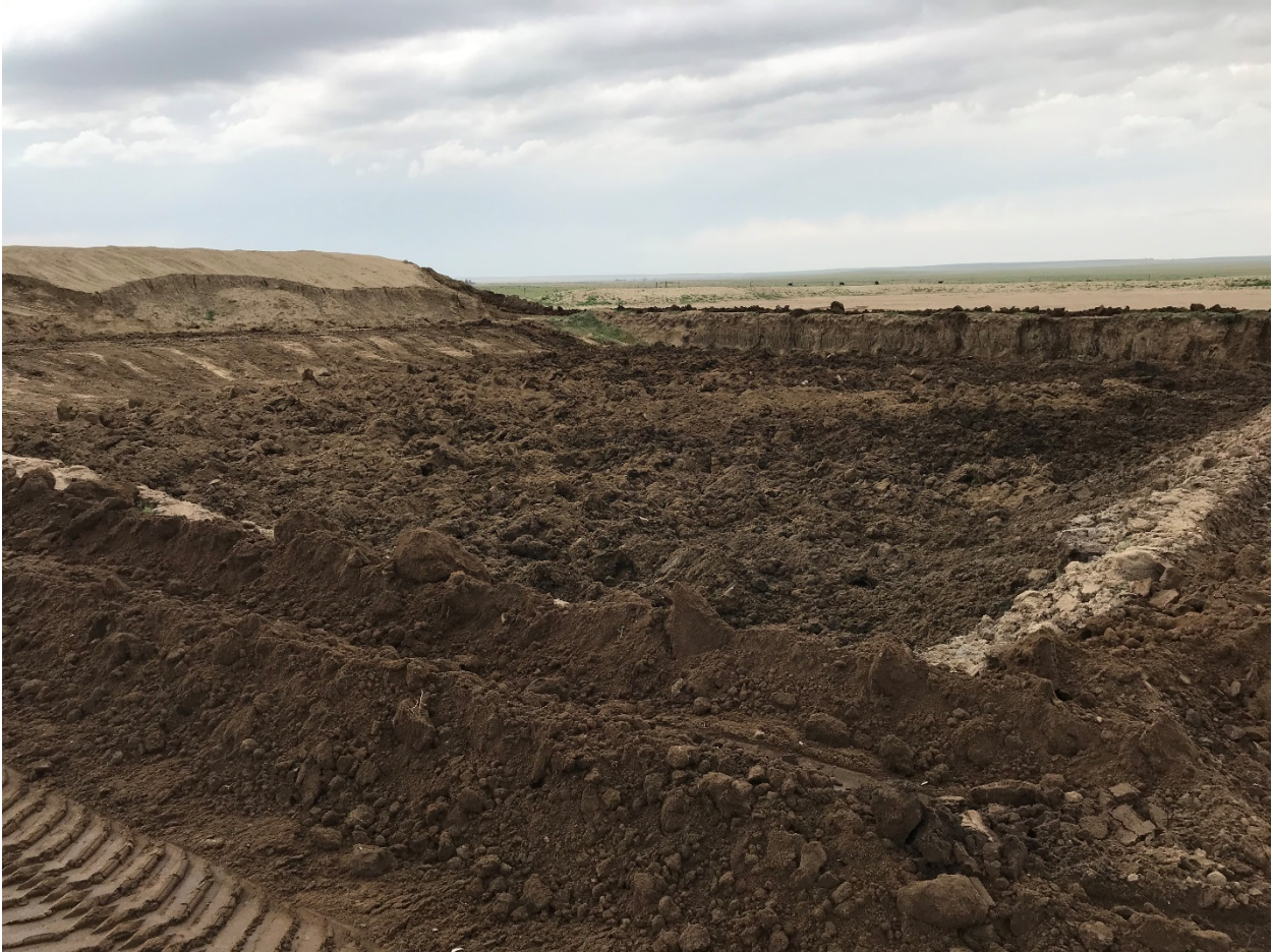
Pit after mixing facing northwest 5/15/21
