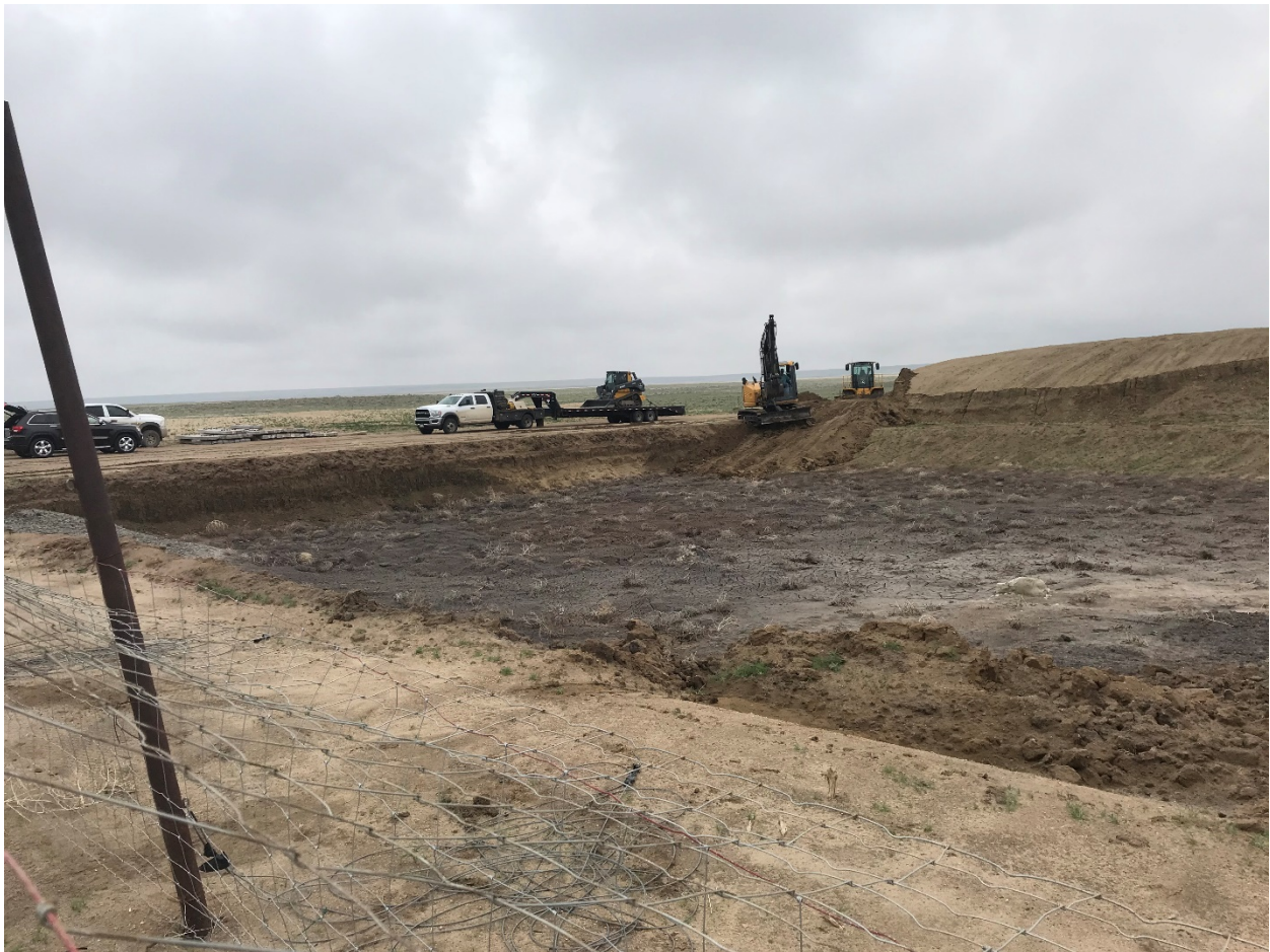
Pit prior to mixing facing southwest 5/15/21
