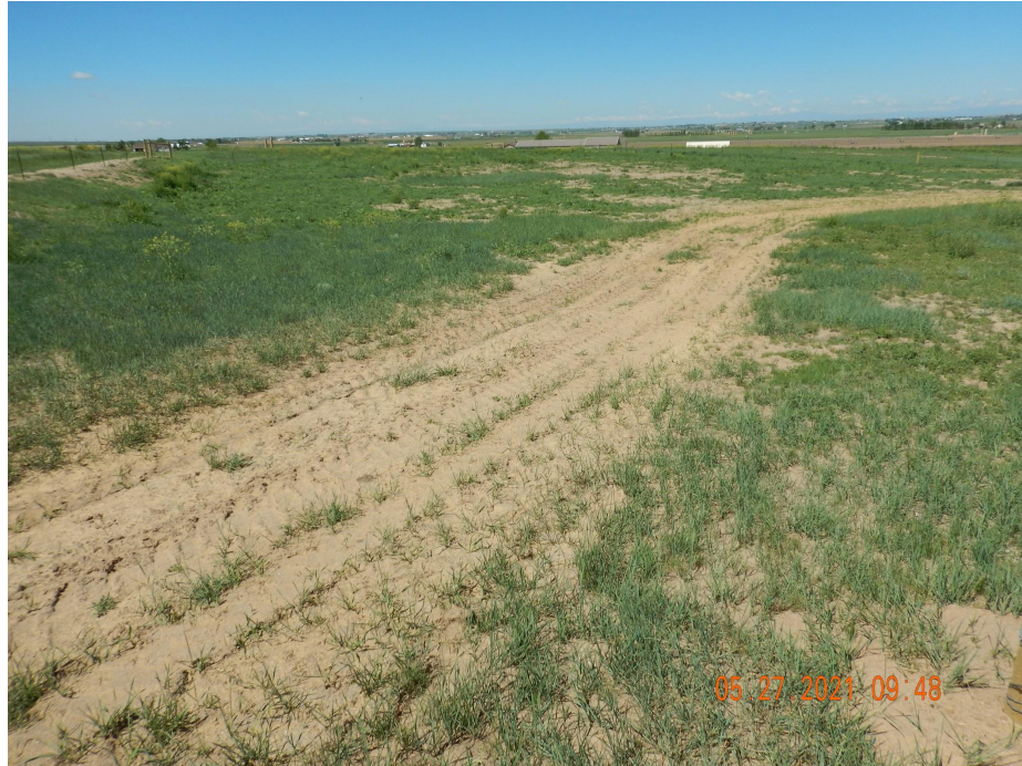
Photo 1. Photo taken from the southeastern well location, facing West. Photo illustrates Operator has fenced off access road and well location. Operator performed interseeding in already established areas that did not have uniform vegetative plant cover. Where there was little or no establishment, Operator seeded and mulched those reclamation areas. Germination of desirable plant species was observed throughout the reclamation areas.
