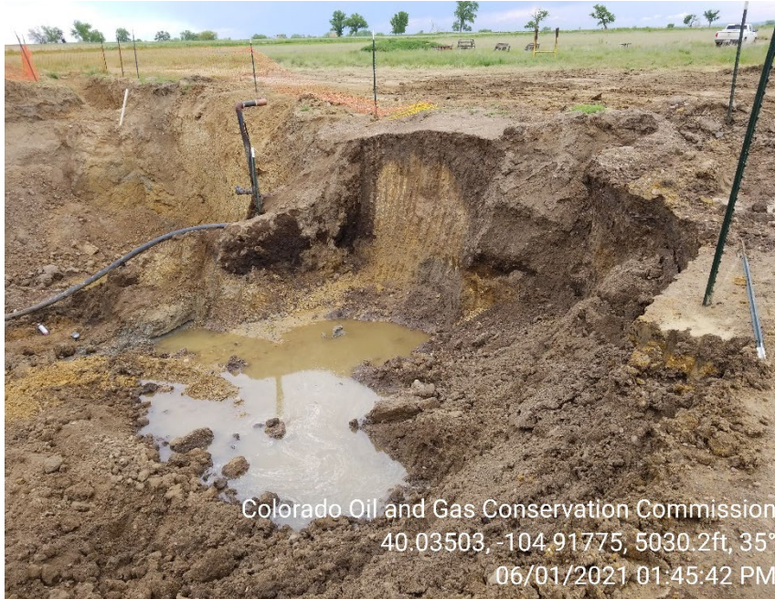
Photo 5 – Open excavation. Impacts remain in situ. Sheen observed on groundwater.
