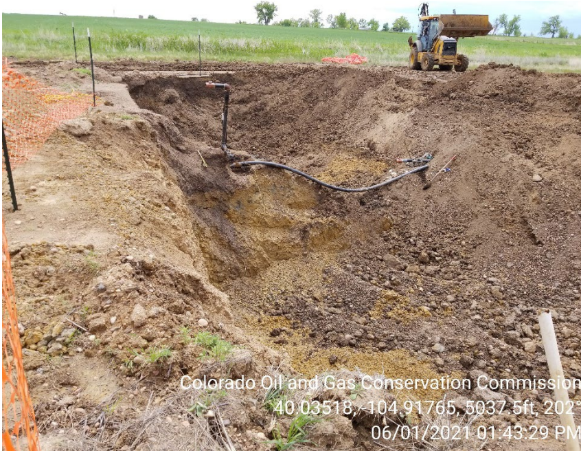
Photo 3 – Open excavation. Area where free product was previously observed appears to have been partially backfilled. Impacts remain in situ.
