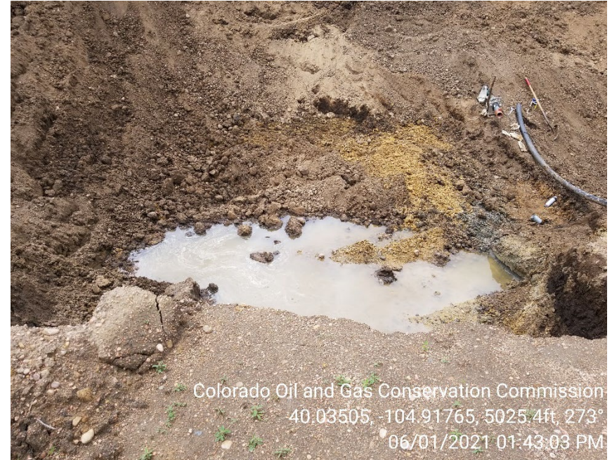
Photo 2 – Expanded area of investigation. Groundwater with hydrocarbon sheen observed. Impacts remain in situ.
