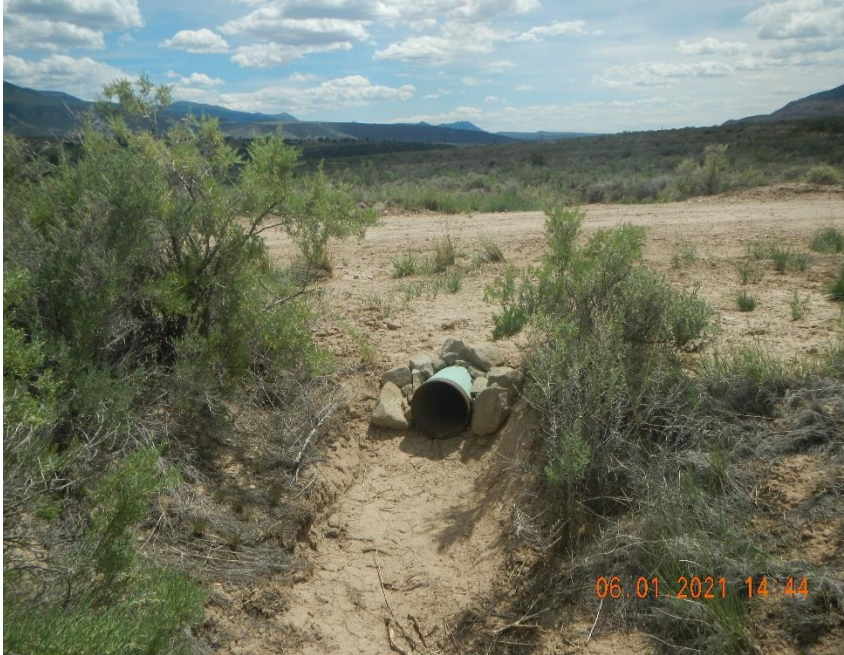
Culvert installed
