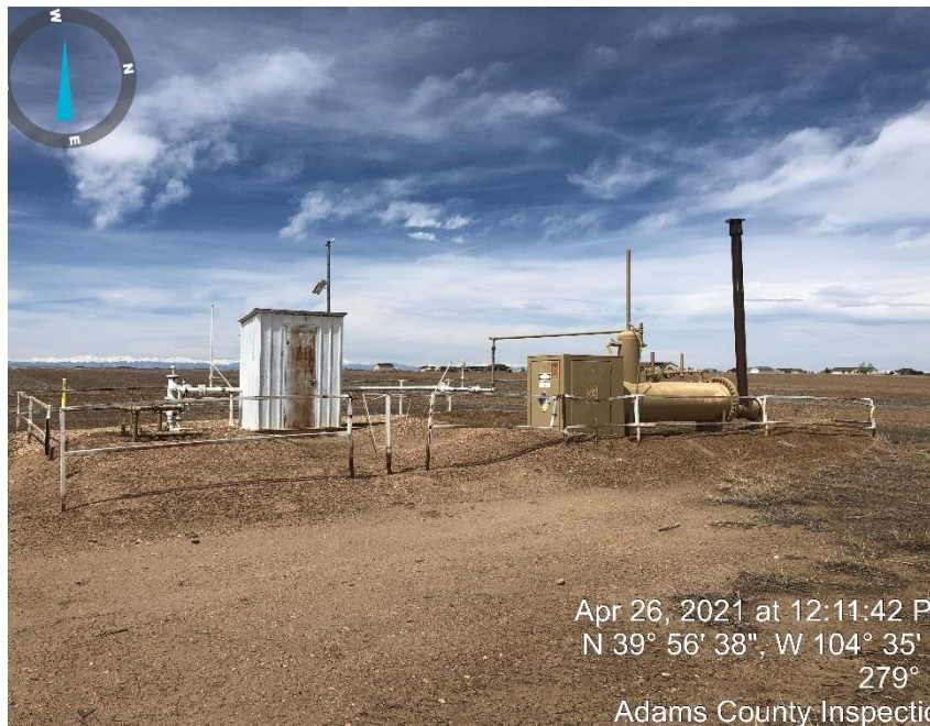
Photo #2 Separator and meter.
