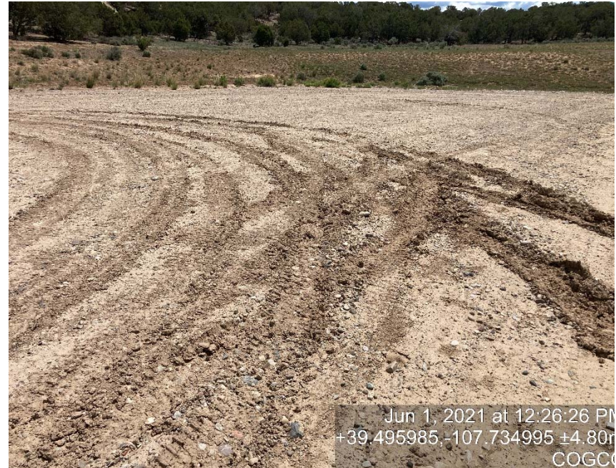
Lack of stabilization/compaction
