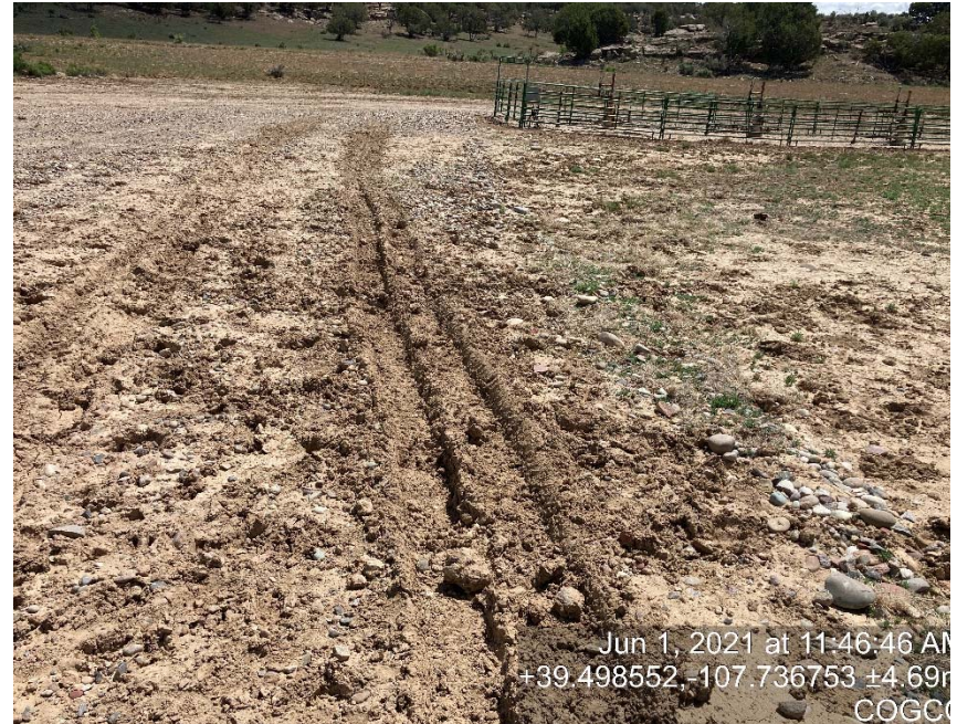
Lack of stabilization/compaction
