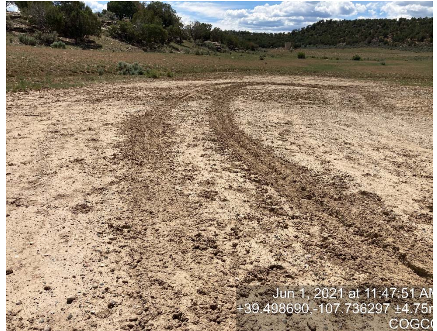
Lack of stabilization/compaction
