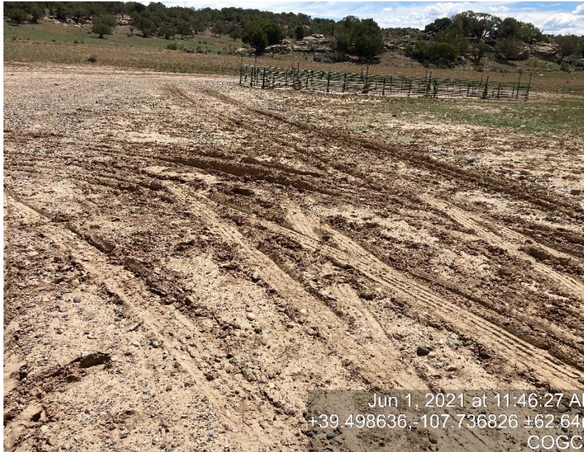
Lack of stabilization/compaction
