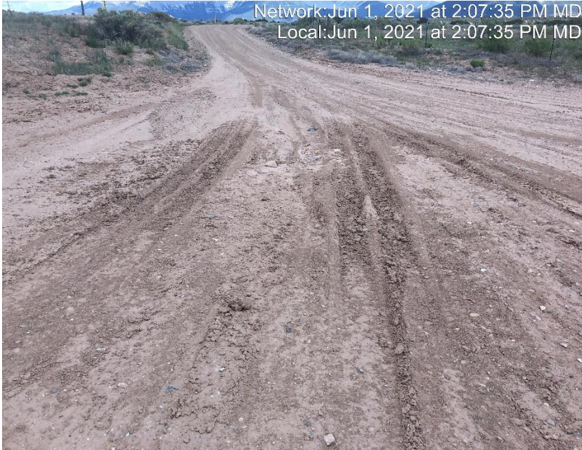
Photo #3995 No form of tracking BMP at entrance to location.
