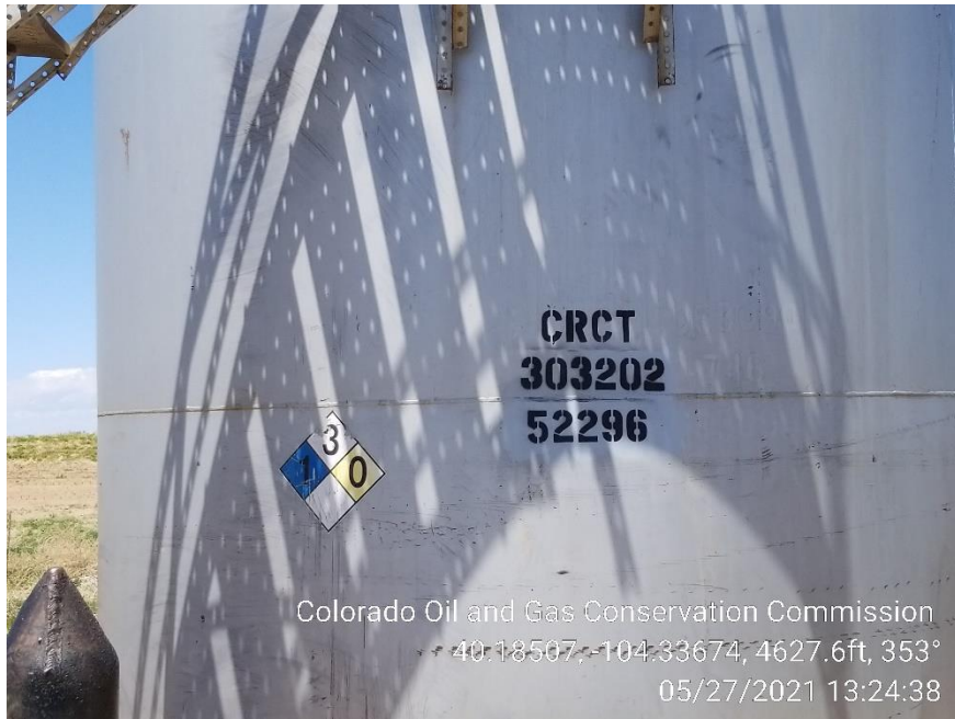
Photo 7 – Content and Capacity Labels missing
