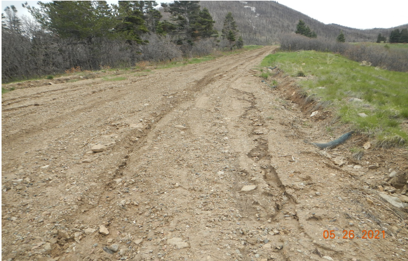
Photo 1. There is erosion occurring down the road ascending to the location. Areas of erosion will need to be repaired and BMP's need maintenance.
