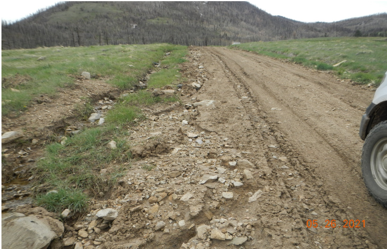
Photo 3. Stormwater is causing erosion along the road near the location.
