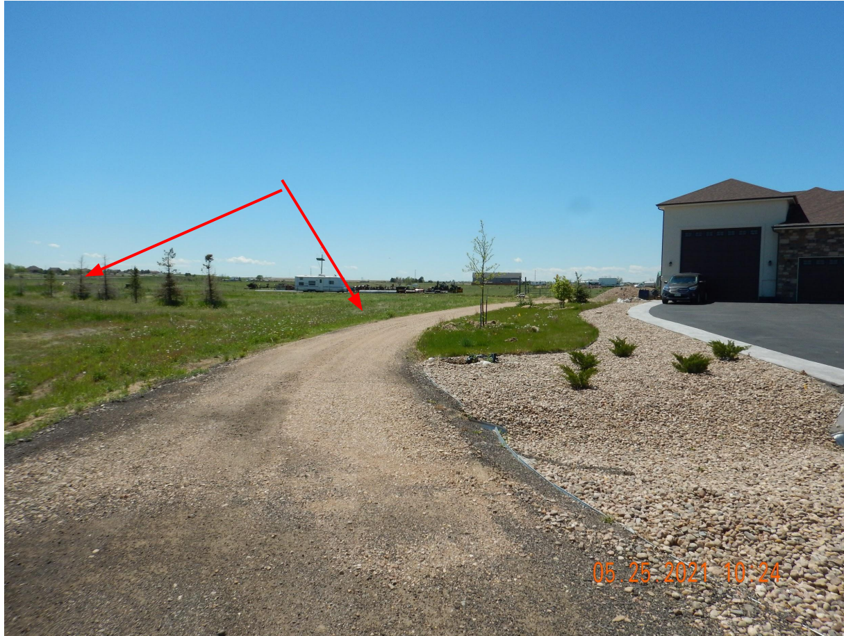
Photo 2. Photo taken from the associated offsite tank battery location, facing South. See comments under Photo 1. Note- the meter house that was previously observed in 2019 has been removed.
