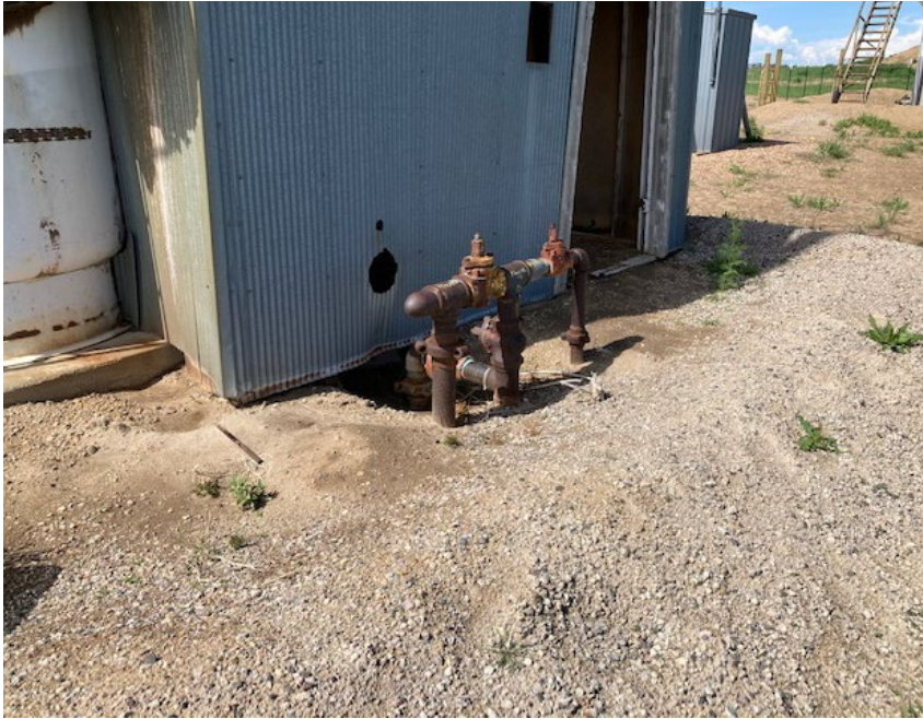
Flow line riser at tank battery
