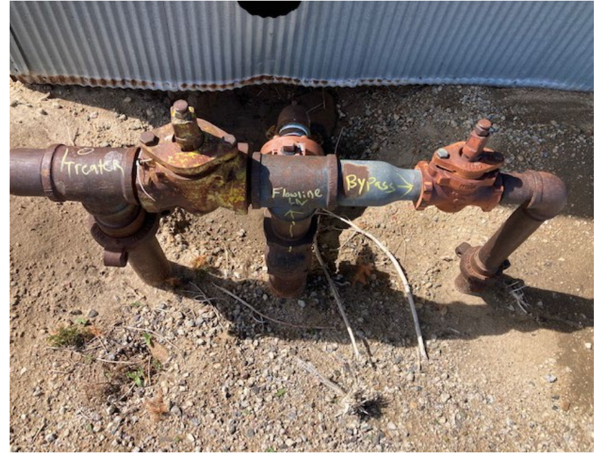
Flow line riser at tank battery
