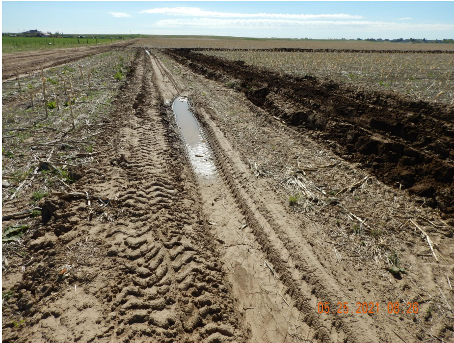
Photo 2. Photo taken from the northern location, facing East. Photo illustrates Operator has installed a ditch and berm BMP around the entire perimeter of the location during construction activities.
