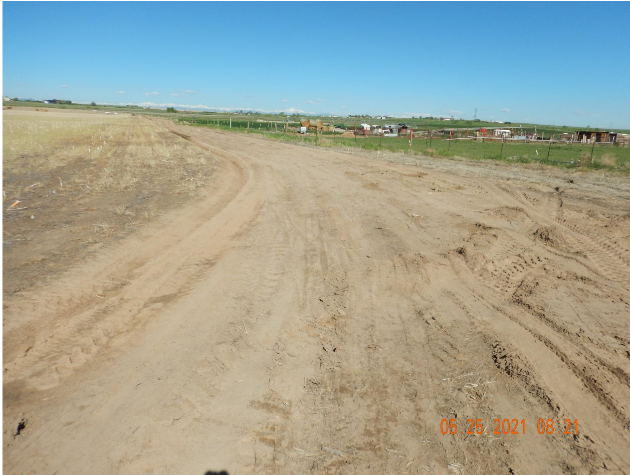
Photo 1. Photo taken from the entrance of location, facing West. Photo illustrates major construction activities have commenced. Operator has installed a ditch BMP along the outer perimeter of the access road.
