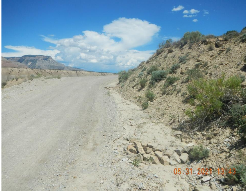
Sediment build up on velocity checks and storm water washing around.
