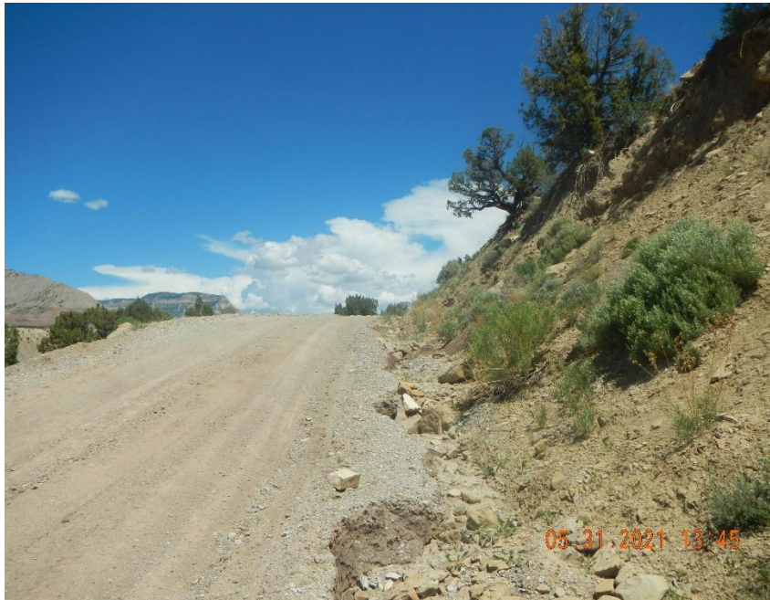
Erosion of road into ditch.
