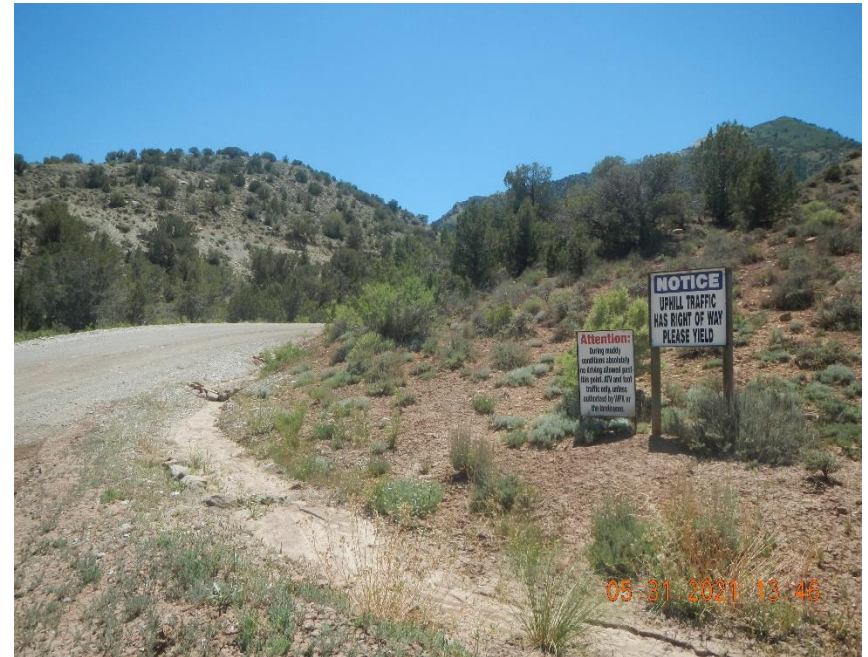
Sediment build up in ditch.
