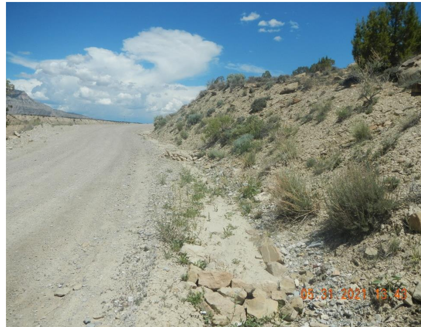
Sediment build up on velocity checks.
