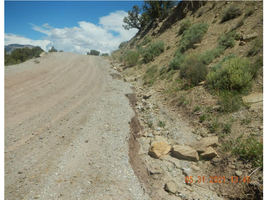
Erosion of road into ditch.
