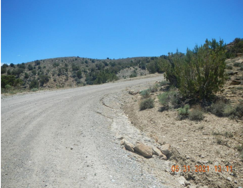
Sediment build up over velocity checks.
