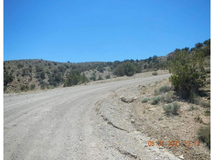
Riling along road ditches.
