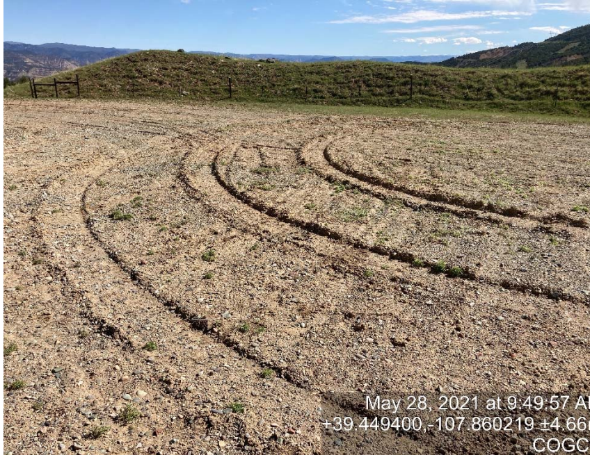
Lack of stabilization/compaction
