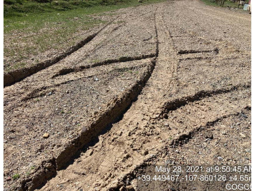
Lack of stabilization/compaction
