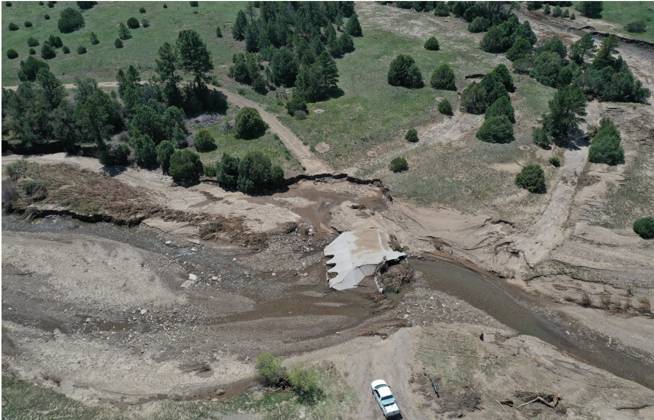
Photo 1. Drone aerial photo facing toward the ephemeral creek crossing where recent flood event has wash out the cement crossing area.
