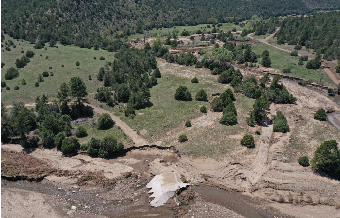
Photo 3. Drone aerial photo facing toward the ephemeral creek crossing where recent flood event has wash out the cement crossing area.
