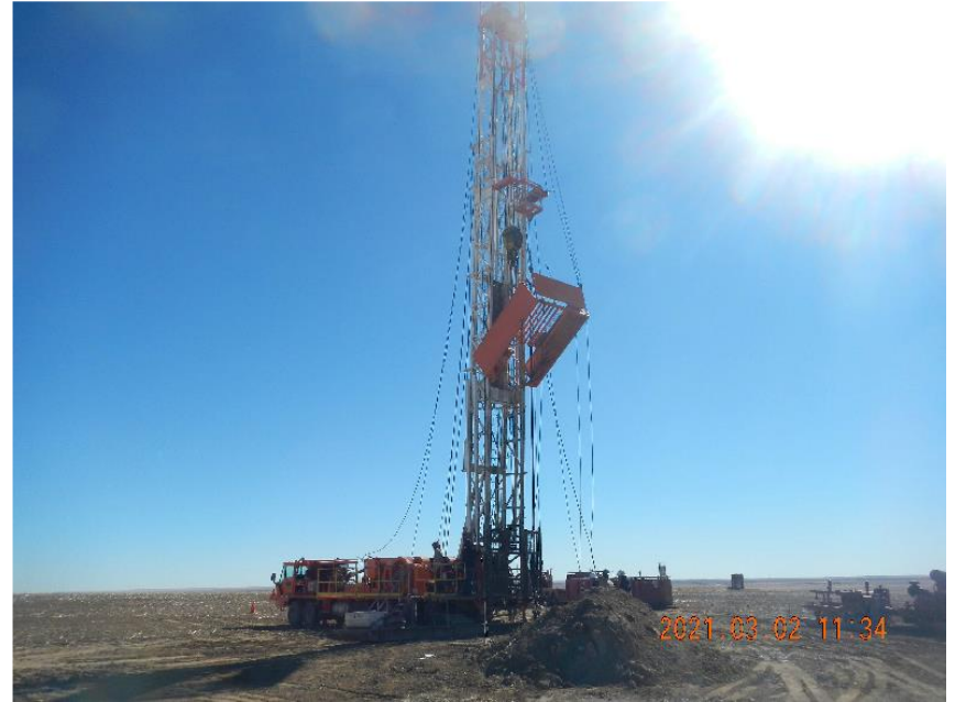
Photo 2: Rig up in progress with mast coming up.
