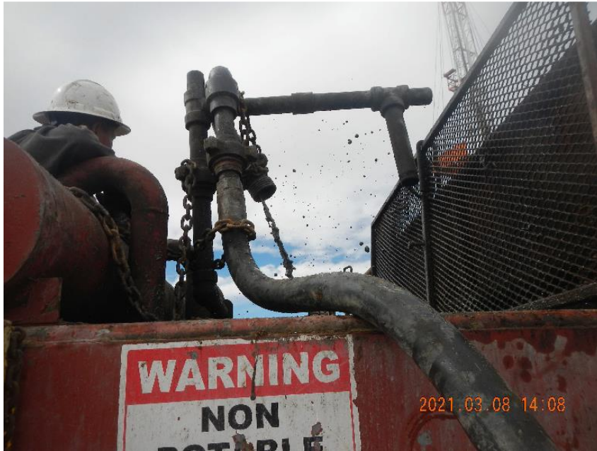
Photo 7: Start of returns while pumping 1 st stage of surface plug.
