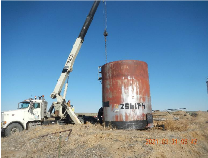
Photo 13: Production tank being lifted for loading and removal.
