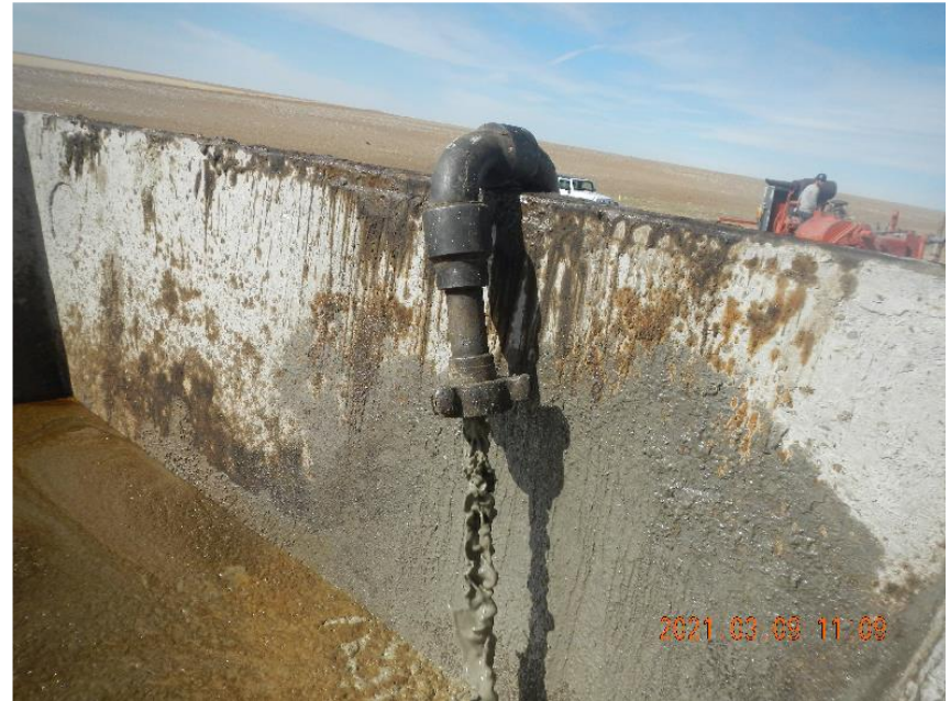
Photo 8: Cement returns to surface pumping final stage of surface plug.
