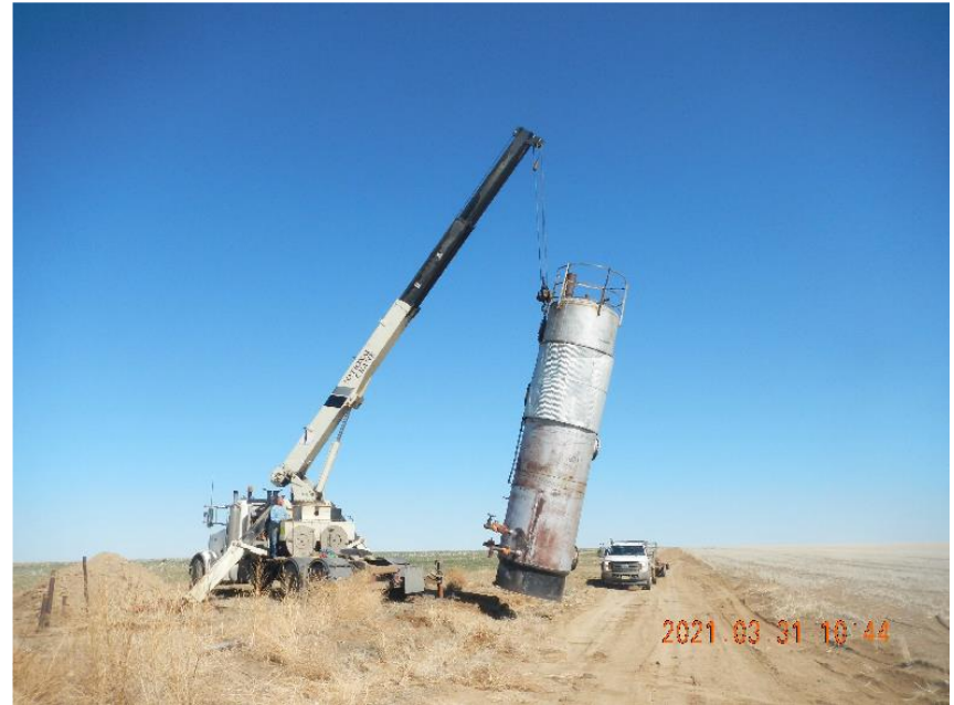
Photo 14: Treater being lifted for loading and removal.
