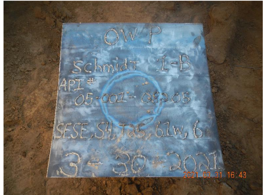
Photo 12: Well cut and capped with marker plate welded onto surface casing.
