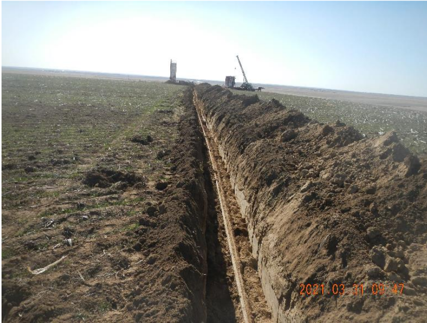
Photo 15: View of trench excavated for flow line removal.
