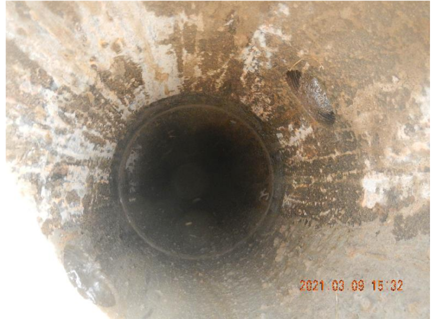
Photo 10: View inside surface casing. Cement tagged at 15' and will be topped off when surface casing is cut off below grade.
