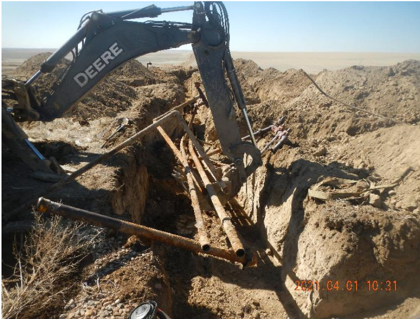
Photo 17: Excavating and removing flow lines at production facility.
