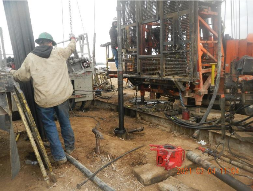
Photo 5: Rig crew pulling production casing out of well after it was cut off.
