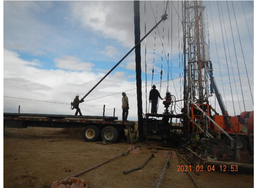
Photo 6: Cut production casing being laid down on flatbed trailer with aid of pipe sling.
