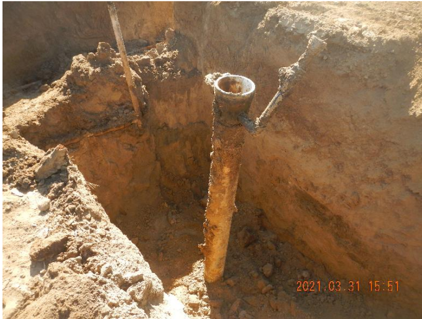
Photo 11: Excavated surface casing.
