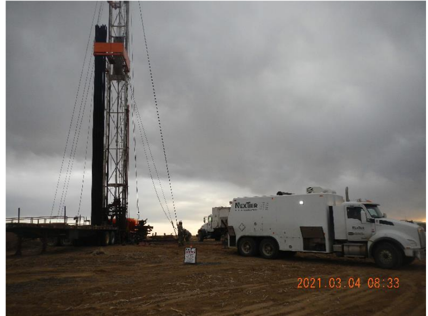
Photo 4: Wireline rigged into well to cut production casing off at 3000'.
