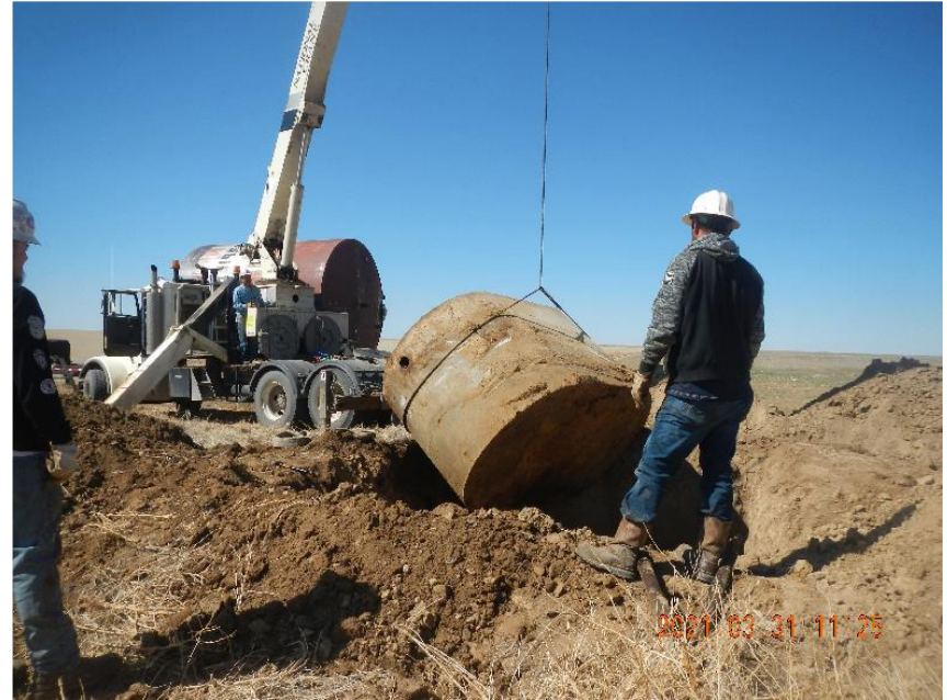
Photo 16: View of excavated produced water vault removal.
