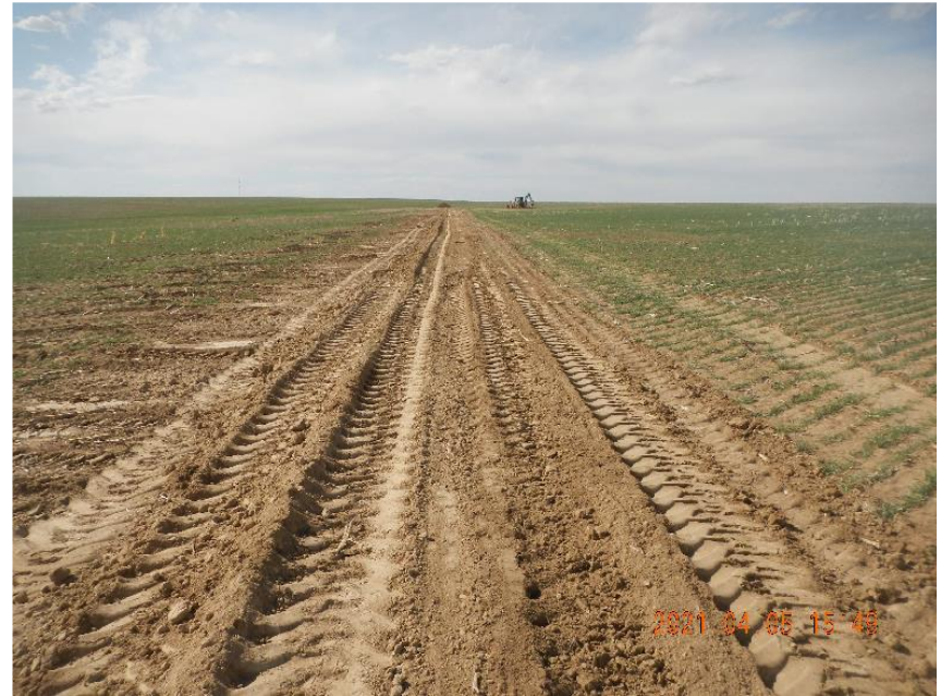
Photo 18: View of backfilled and dressed flow line trench.
