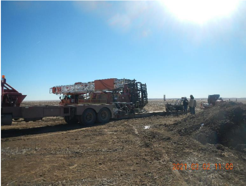
Photo 1: Rig spotted in over wellhead.
