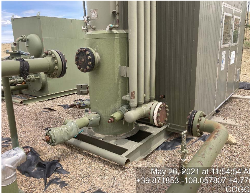
Dehy not connected (unused equipment)
