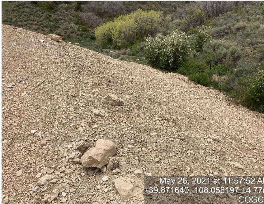
Fill slope not stabilized
