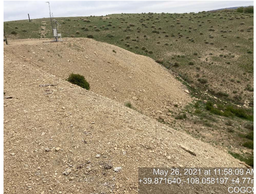
Fill slope not stabilized
