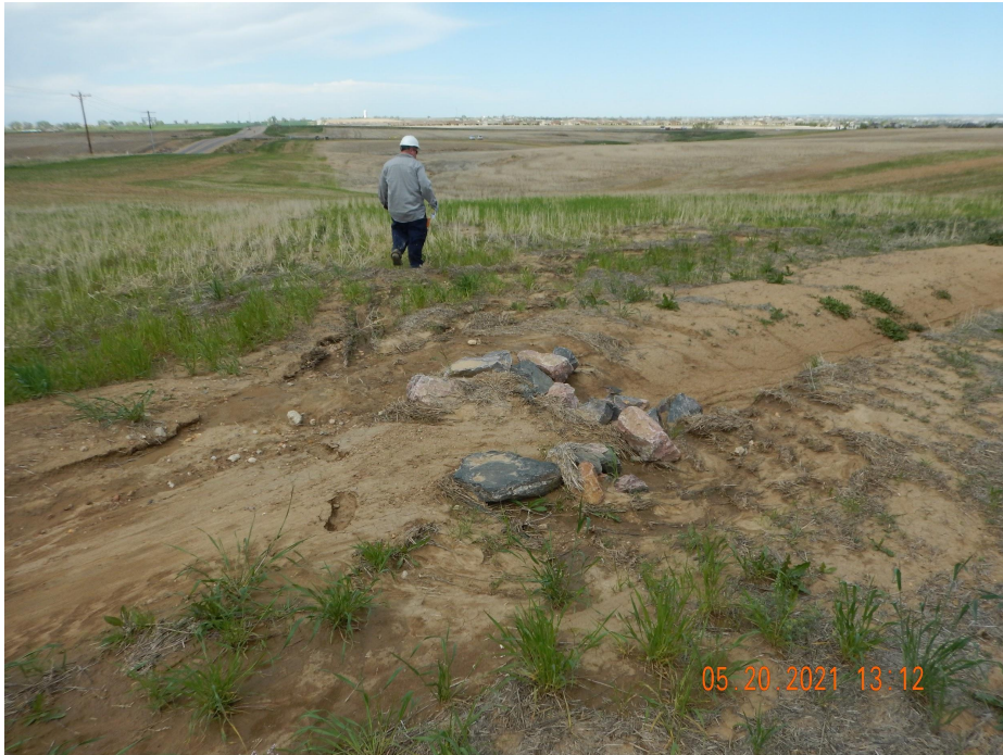
Photo 7. Photo taken from the northwestern location, facing North. Photo illustrates sediment has filled up the check dam and is discharging sediment offsite.
