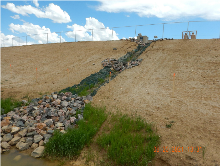
Photo 11. Photo taken from the northeastern location, facing South. Photo illustrates a stabilized channel with check dams and appears maintenance is required along the upslope portion.
