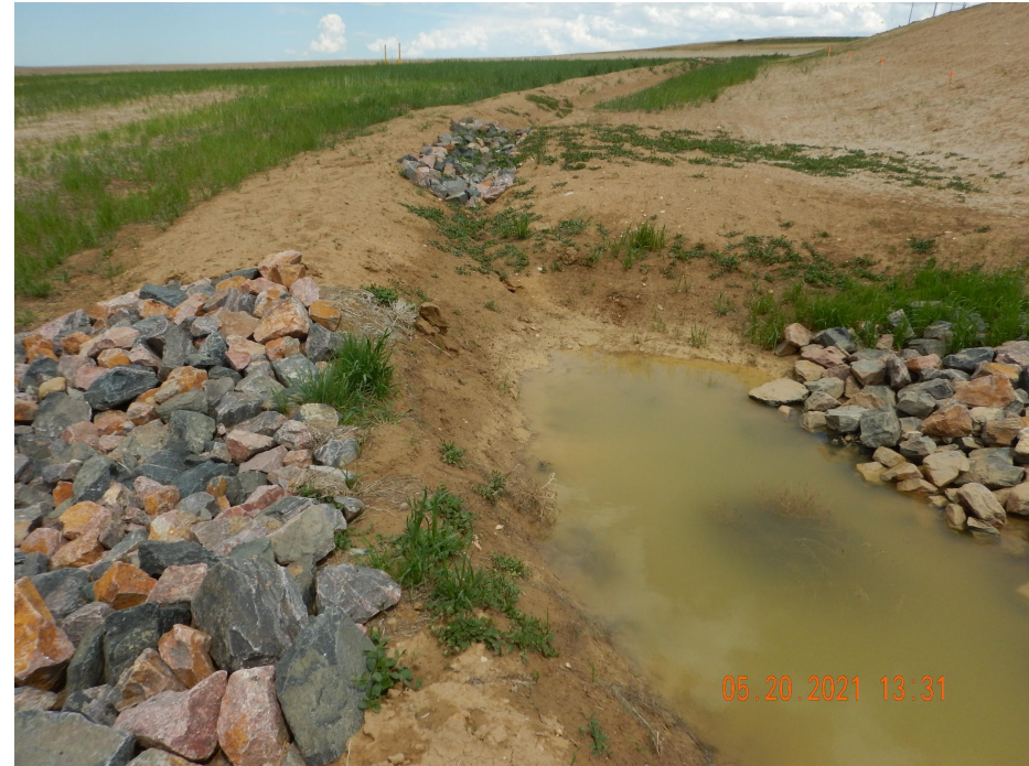
Photo 12. Photo taken from the northeastern location, facing East. Photo illustrates a sediment trap in need of maintenance.
