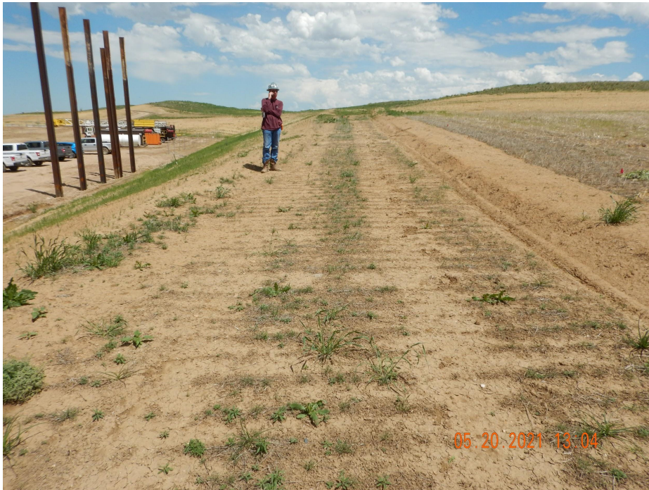
Photo 1. Photo taken from the southern location, facing East. Photo illustrates a ditch BMP along the perimeter with the cut slope to the interior.
