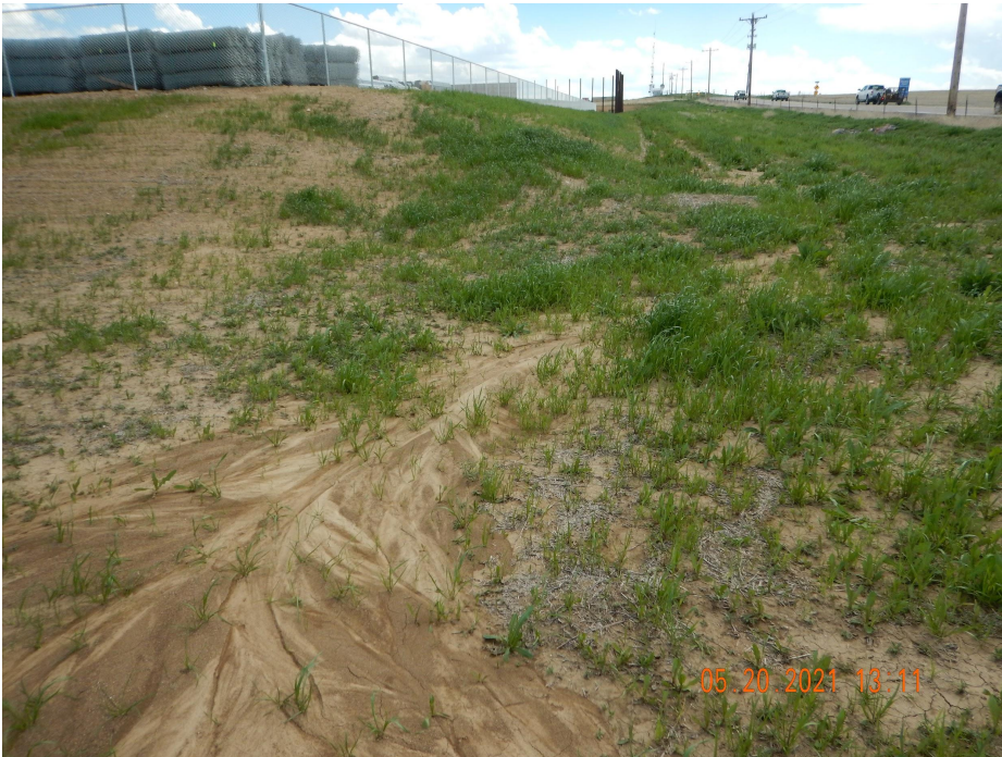
Photo 5. Photo taken from the northwestern location, facing South. Photo illustrates a path of erosion.
