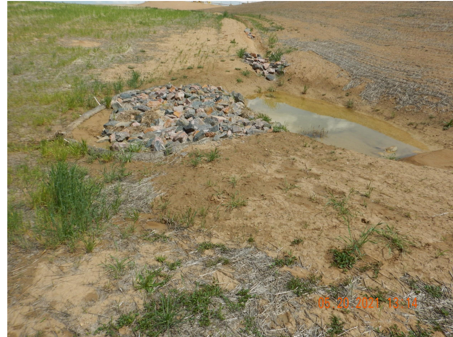
Photo 10. Photo taken from the northern location, facing East. Photo illustrates a sediment trap in need of maintenance.
