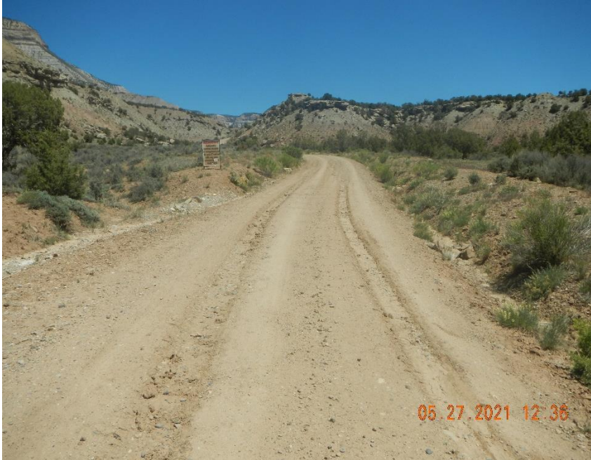
Rutting on access road up to location.
