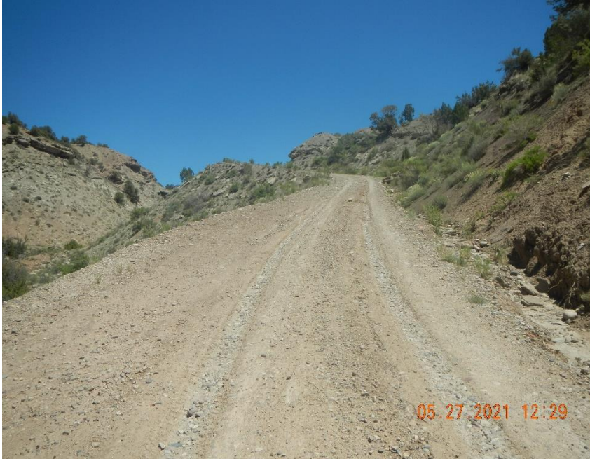
Rutting on access road up hill to location.
