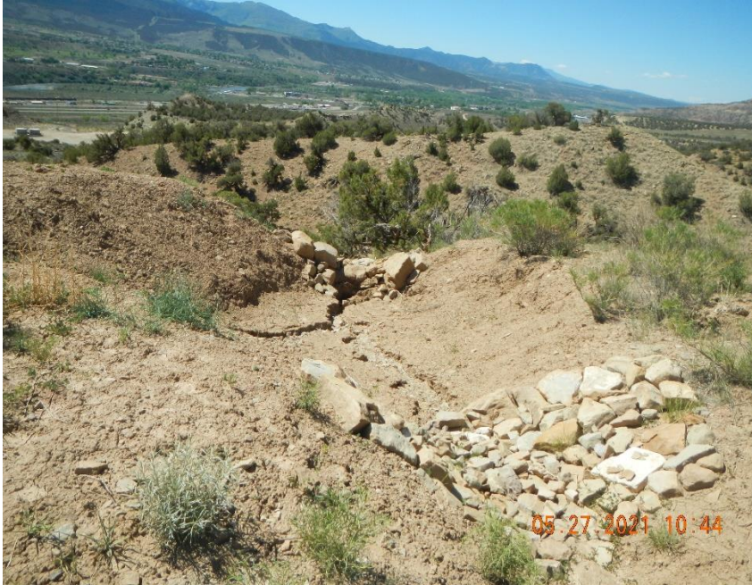
Check dam at south end of location.
