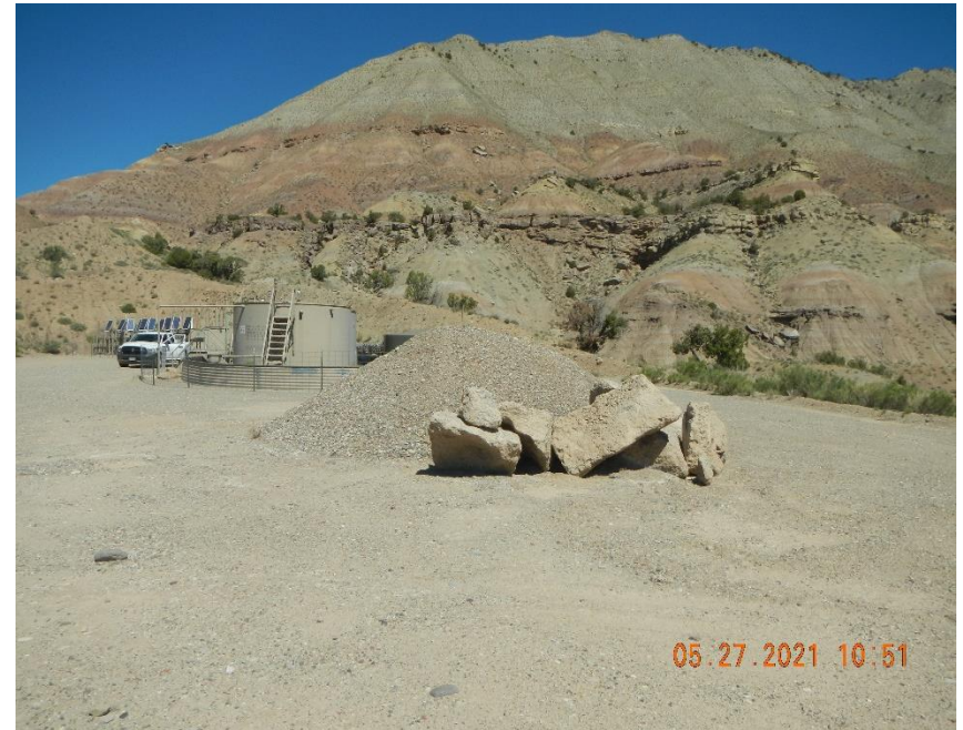
Stock pile with no berm.
