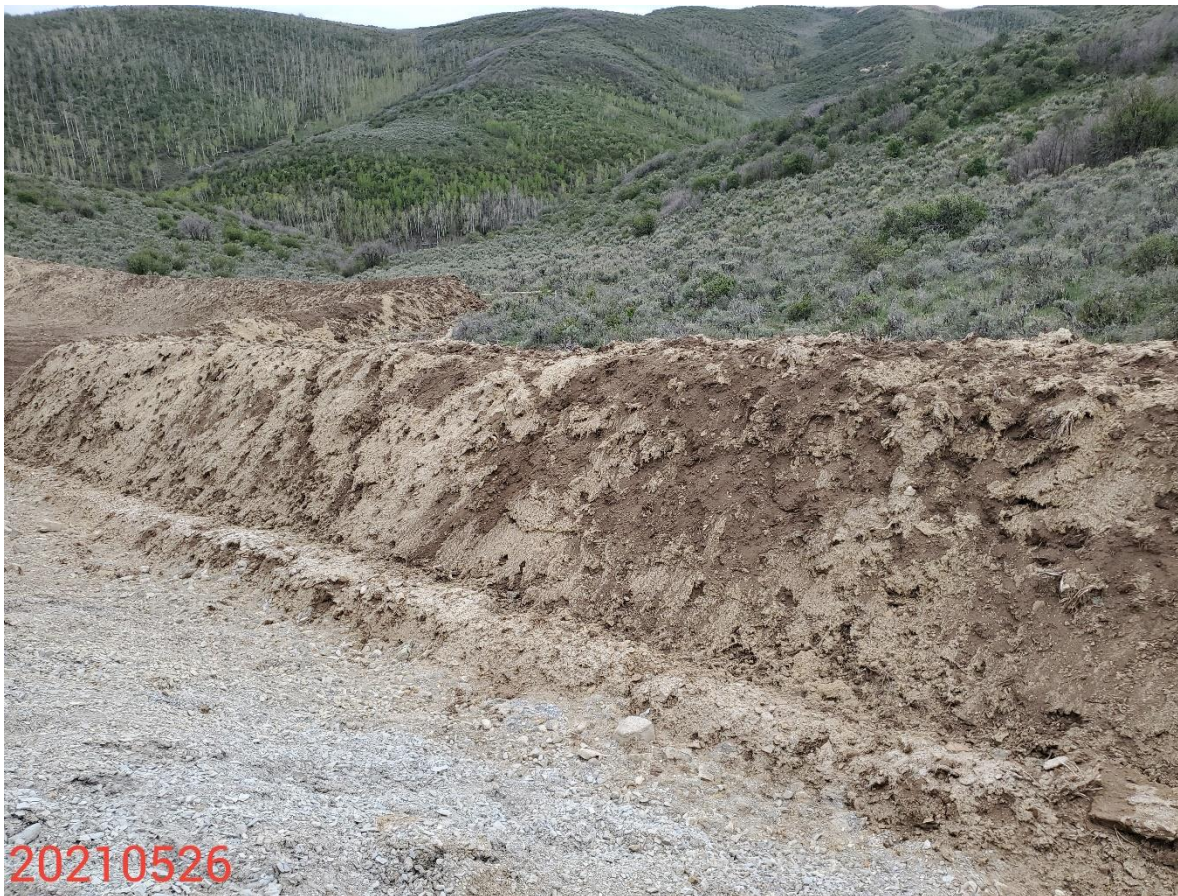
Photo 8: Photo taken from the west end of the Location, facing southwest. Photo show Operator has utilized topsoil at the base of the fill slopes/subsoils of the Location as a berm and sediment trap/pond to manage stormwater; topsoil at risk of degradation, loss and displacement due to stormwater discharge. Photo also shows hydromulch on soils is no longer in proper functioning condition.
