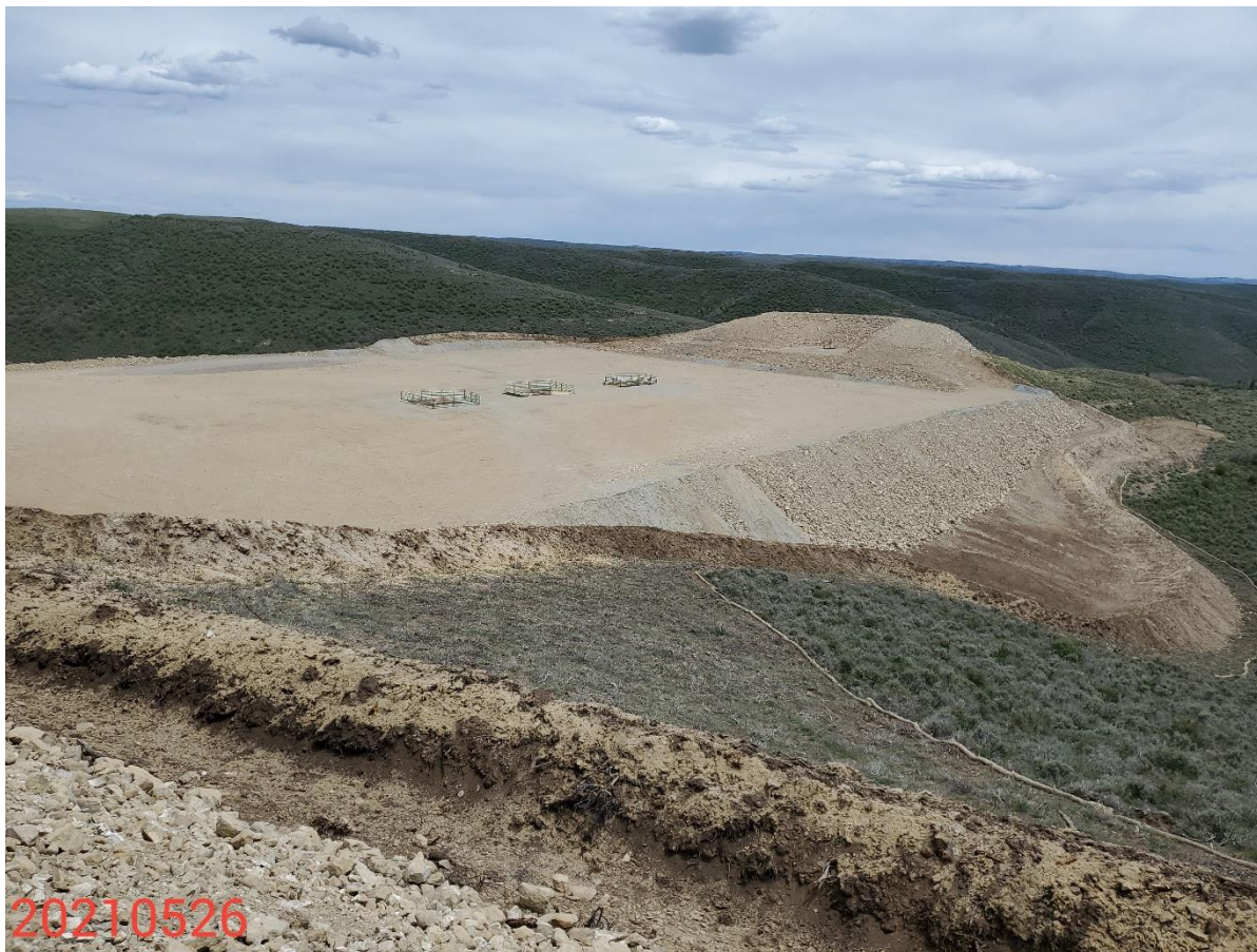
Photo 2: Photo taken from the south end of the frac pad, facing southeast. Photo provides an overview of the Location. Photo also shows Operator has utilized topsoil at the base of the fill slopes/subsoils of the Location as a berm and sediment trap/pond to manage stormwater; topsoil at risk of degradation, loss and displacement due to stormwater discharge
