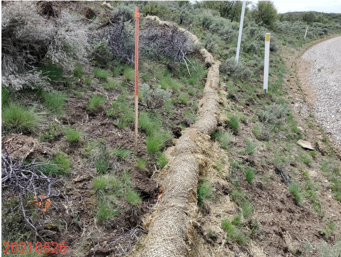
Photo 12: Photo shows examples of erosion logs observed that are either not installed in accordance with good engineering practices, or maintained in a proper functioning condition; wattles not trenched/backfilled.
