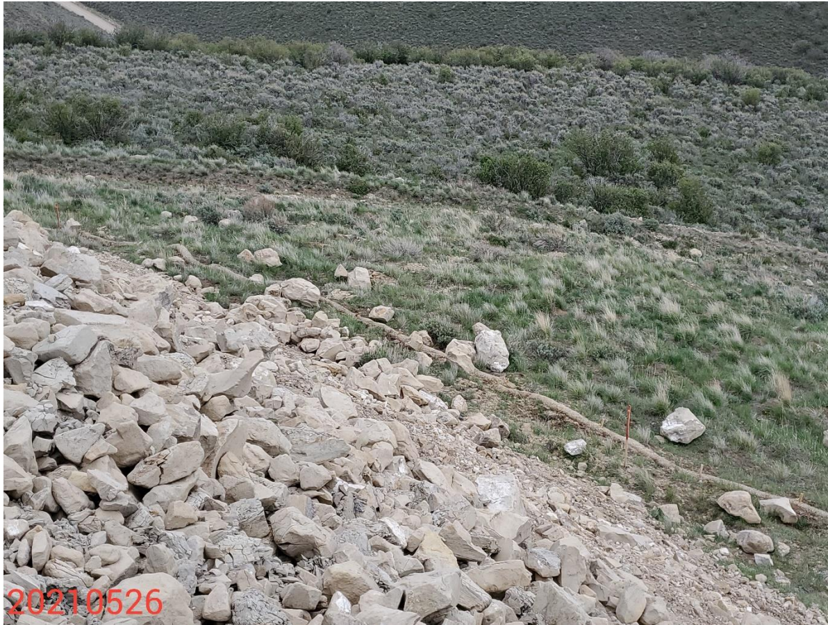
Photo 6: Photo shows control measures to protect/stabilize the cut/fill slopes of the Location is missing or insufficient.
