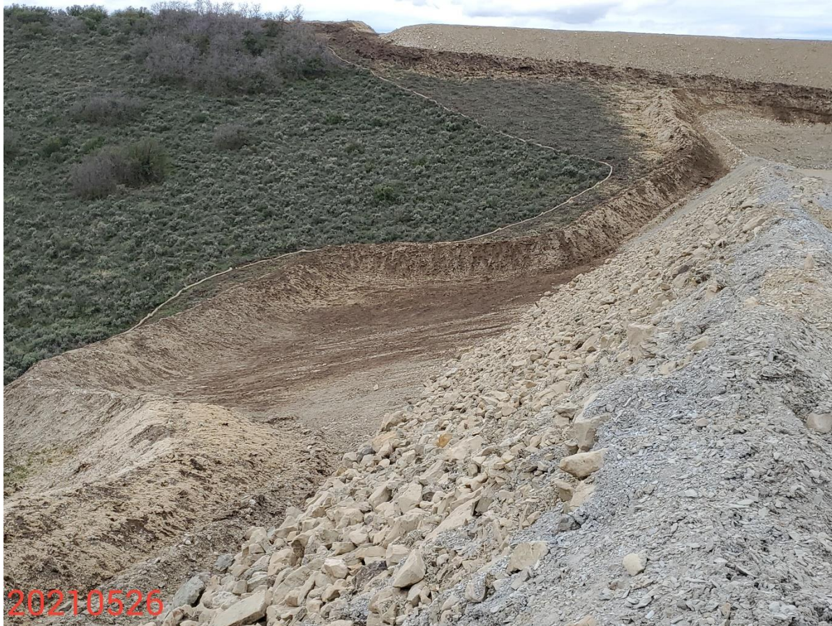
Photo 7: Photo taken from the west end of the Location, facing northwest. Photo shows Operator has utilized topsoil at the base of the fill slopes/subsoils of the Location as a berm and sediment trap/pond to manage stormwater; topsoil at risk of degradation, loss and displacement due to stormwater discharge
