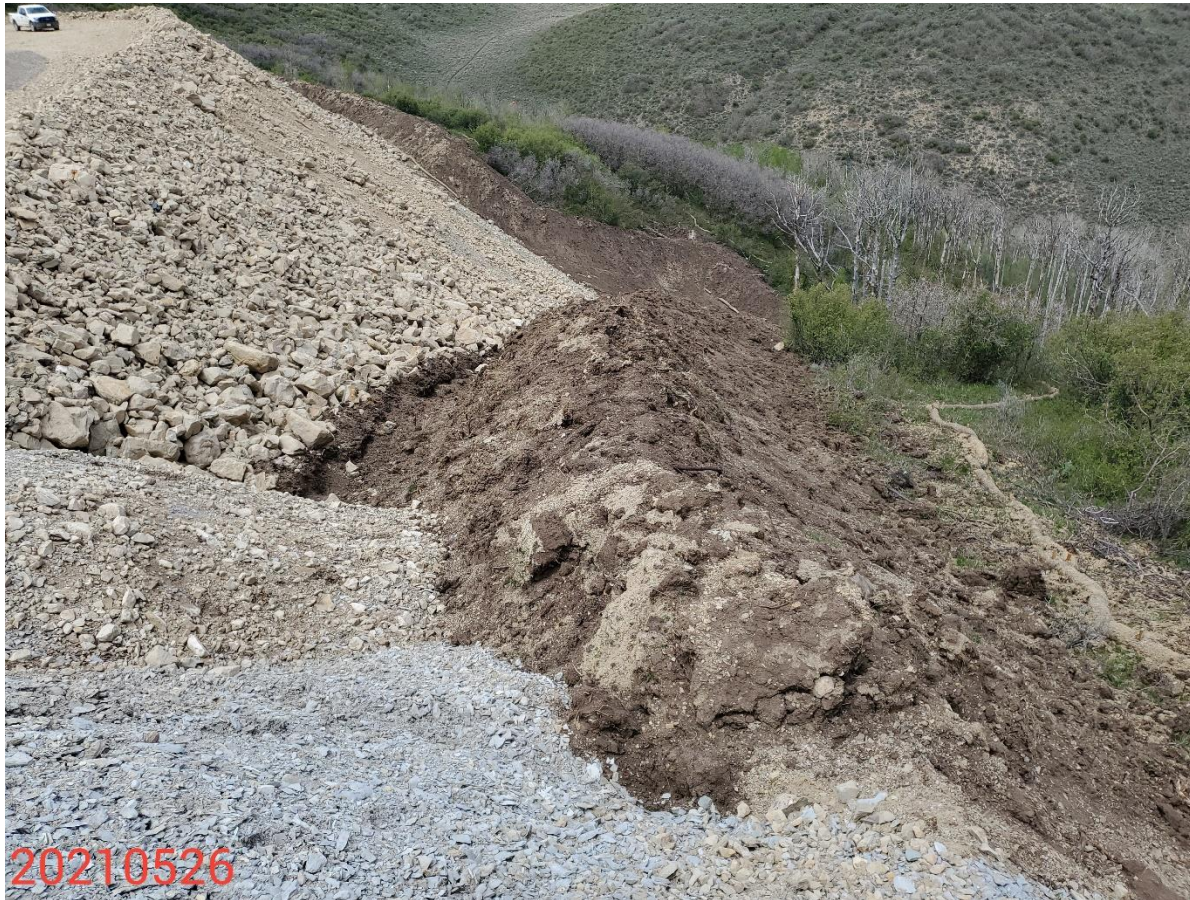
Photo 3: Photo taken from the east end of the Location, facing north. Photo show Operator has utilized topsoil at the base of the fill slopes/subsoils of the Location as a berm and sediment trap/pond to manage stormwater; topsoil at risk of degradation, loss and displacement due to stormwater discharge. Photo also shows hydromulch on soils is no longer in proper functioning condition.
