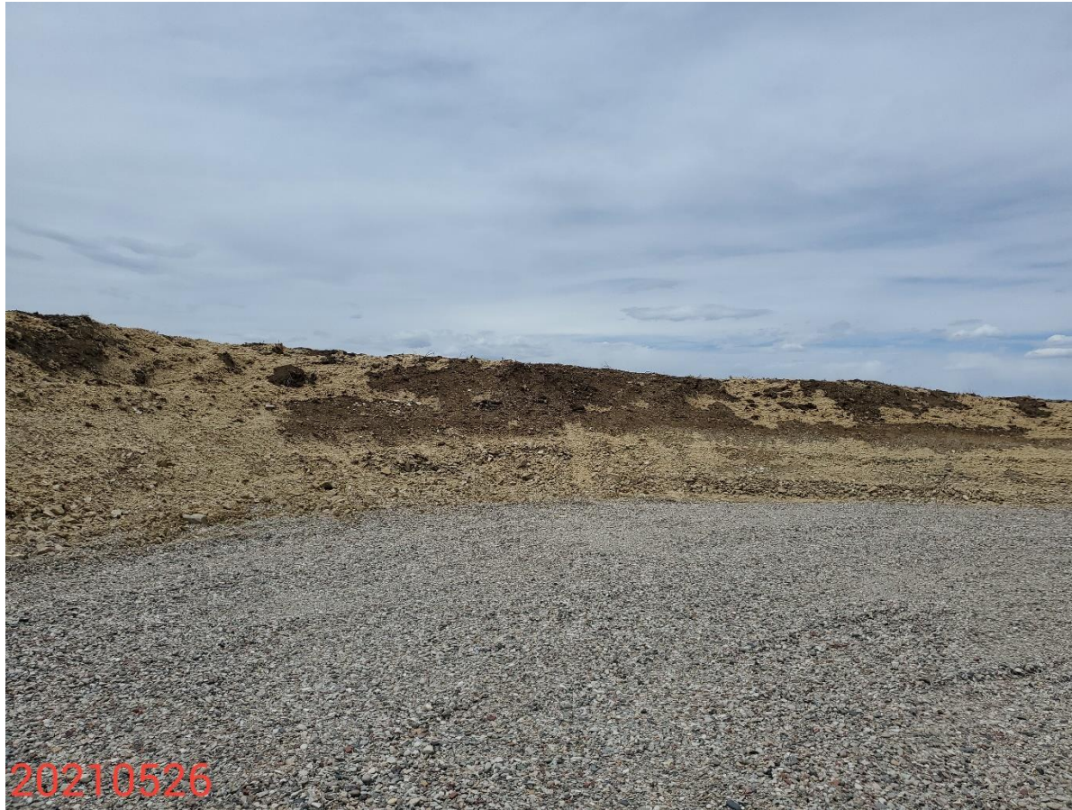
Photo 14: Photo taken from the frac pad, facing northwest. Photo shows hydromulch on soils is no longer in proper functioning condition.
