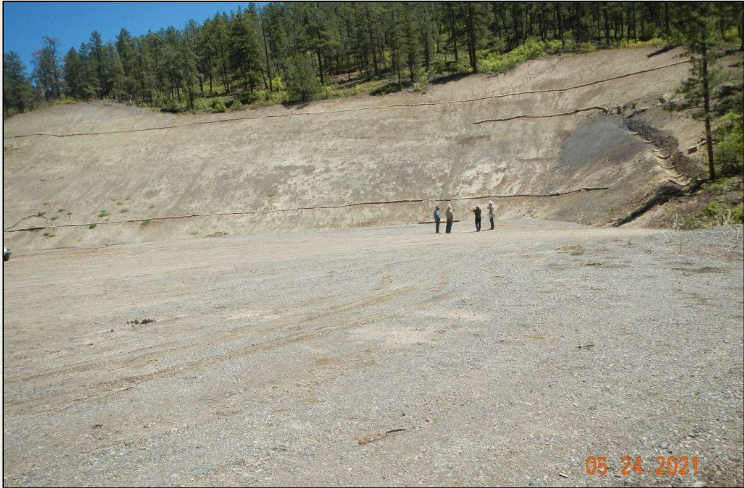
Photos 3. View of the eastern cut-slope. Operator and USFS discussed long term stabilization measures including construction of a ditch, seeding with three different hydro mulch compositions, and erosion control blankets.
