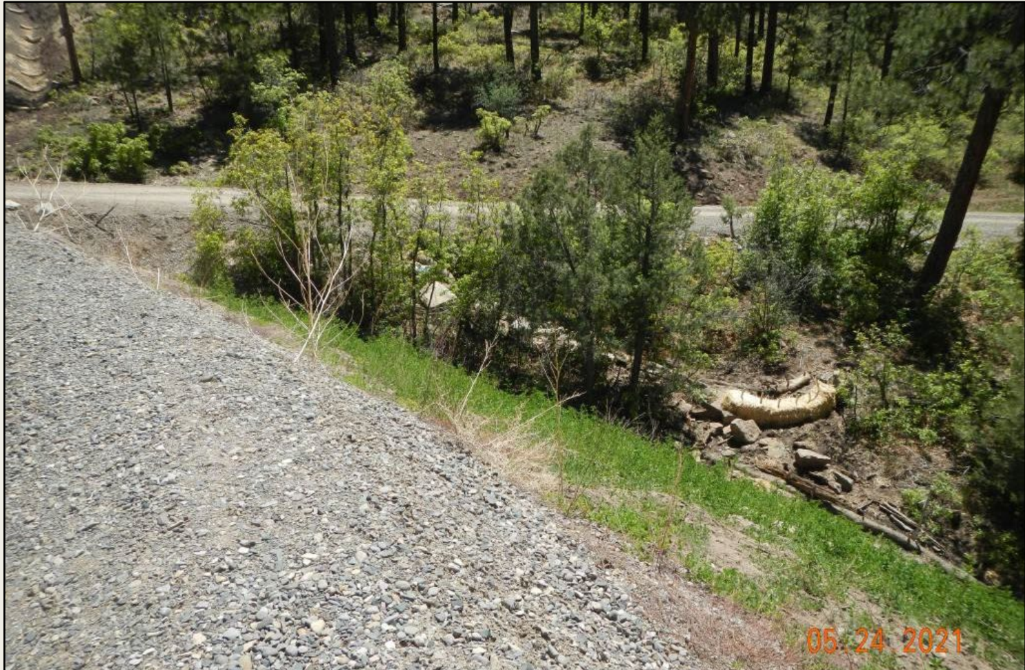
Photo 4. View of area at well pad entrance where concentrated stormwater flows out of a culvert and downslope toward a drainage exiting the western edge of the project area. Operator and USFS discussed installing an extended rock apron here and rock checks along erosional channeling (stormwater flowline) downslope.
