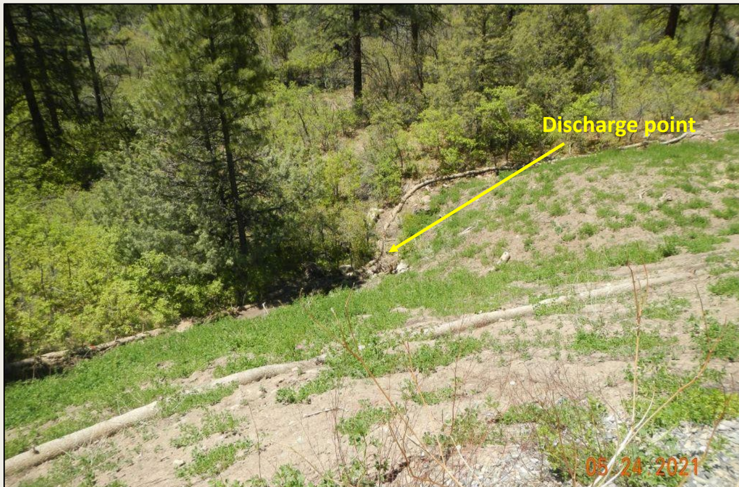
Photo 5. View of discharge point for the well pad and cut-slope into an ephemeral drainage. Operator and USFS discussed installation of an armored silt trap and discharge point here.
