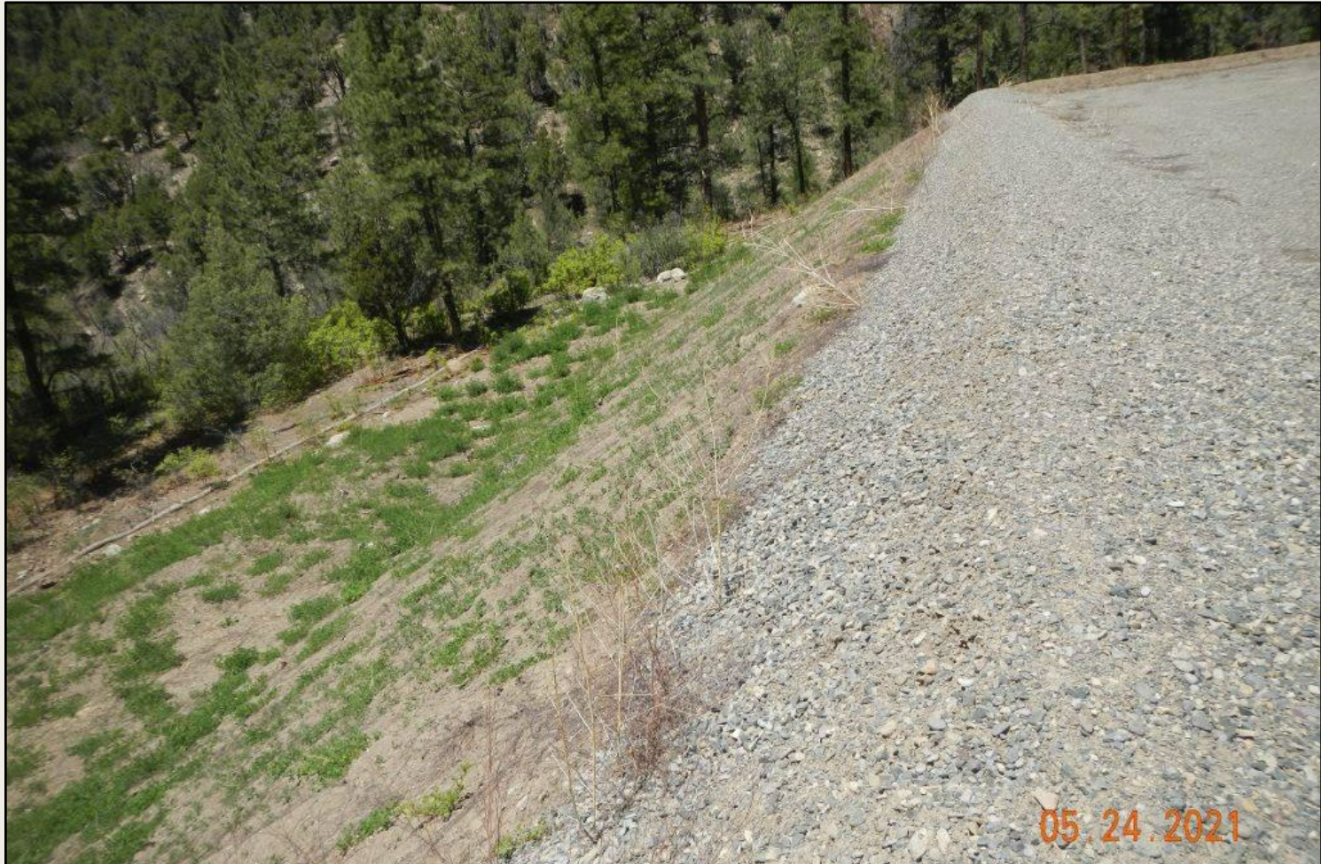
Photo 2. View of the northern project area from the northwestern corner facing westward. Revegetation is sparse. Operator discussed need to conduct spot seeding within the interim reclamation areas.
