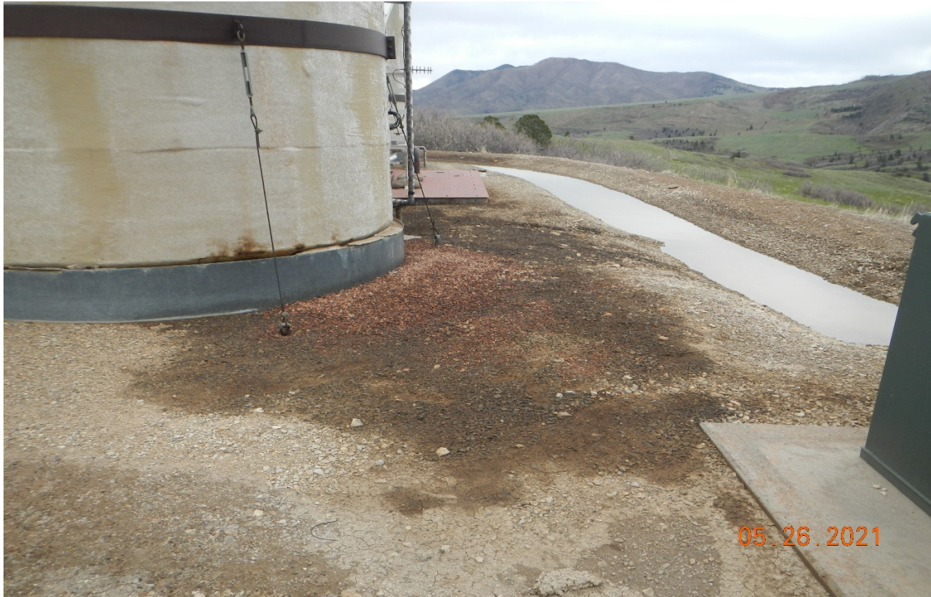
Photo 5. The oil stained soils near the tank need to be cleaned up.
