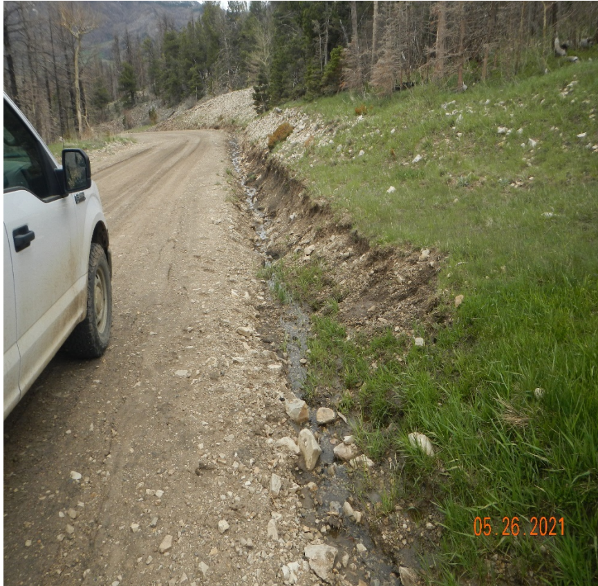
Photo 1. There is an area along the side of the road that is eroding Lat/Long:37.66008, -105.18761.
