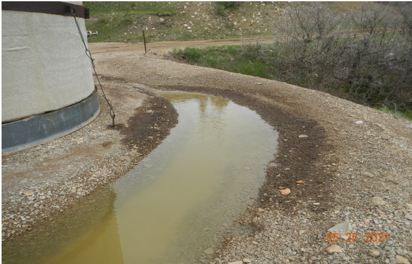
Photo 6. The oil staining appear to have been contained inside the bermed area.
