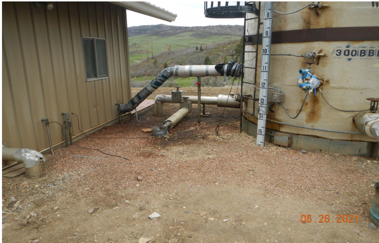
Photo 4. There oil stained soil near the tank battery. This issues was previously observed before and there maybe a mechanical issue causing the leak to occur.
