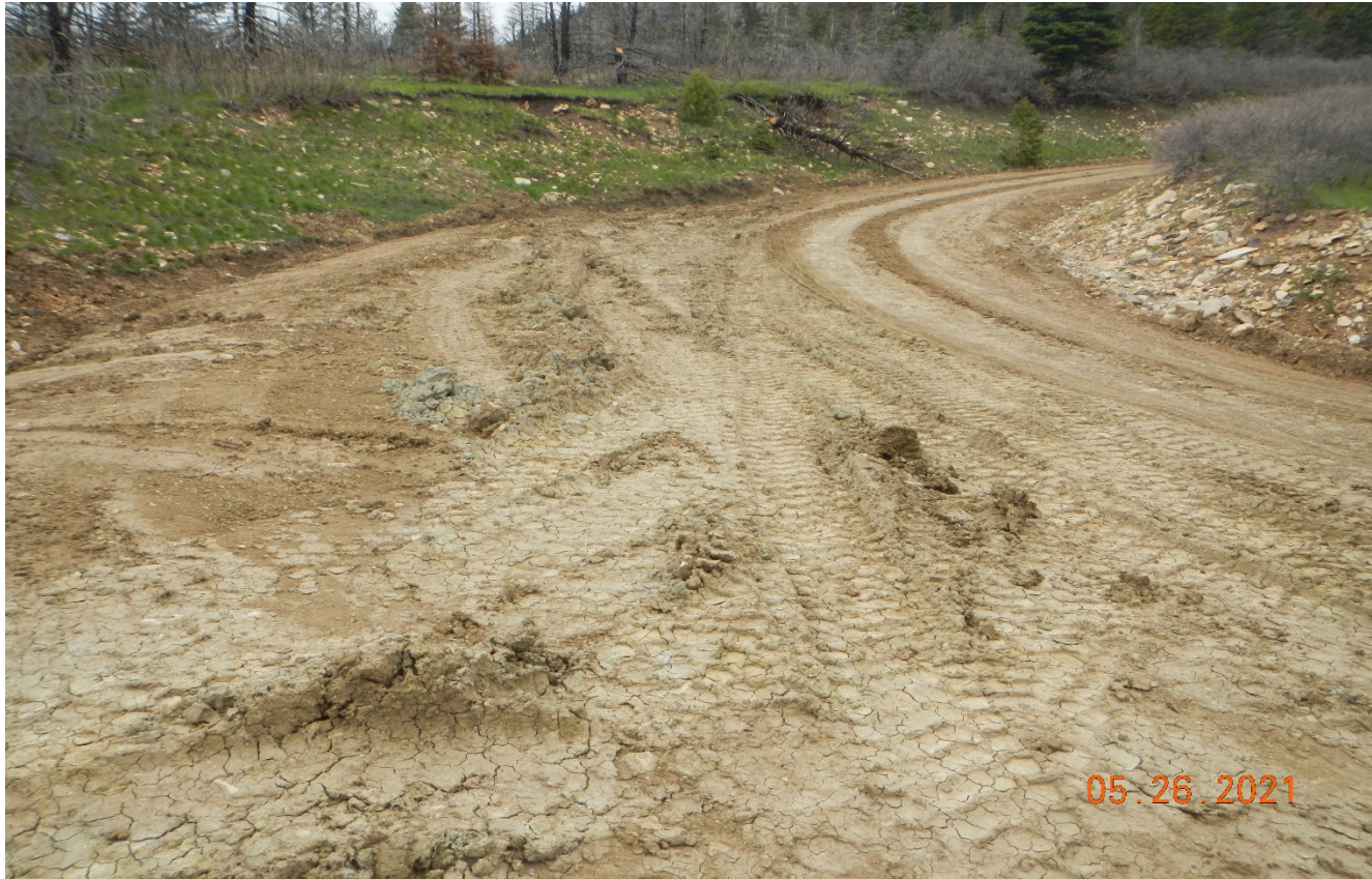
Photo 2. It appears there was a recent high precipitation event that caused issues on the road. It appear the road was in process to be fixed but was not yet completed.
