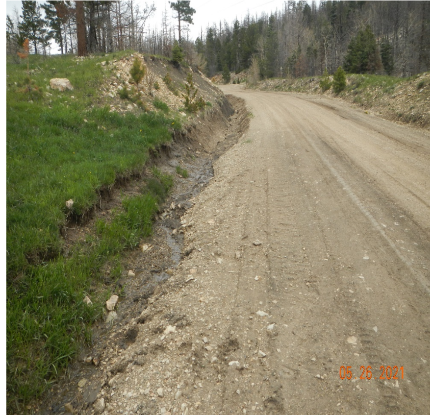
Photo 1. There is an area along the side of the road that is eroding Lat/Long:37.66008, -105.18761.
