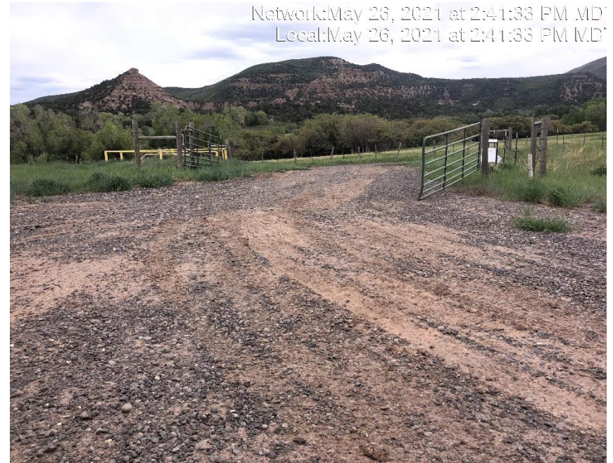
Photo #3958 No form of tracking BMP located at the entrance to location.
