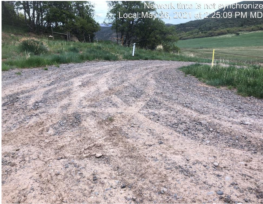
Photo #3952 No form of tracking BMP located at entrance to location.
