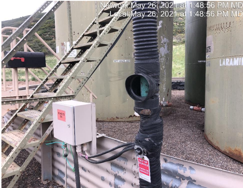
Photo #3943 Flow line heating insulation open ended and not capped.
