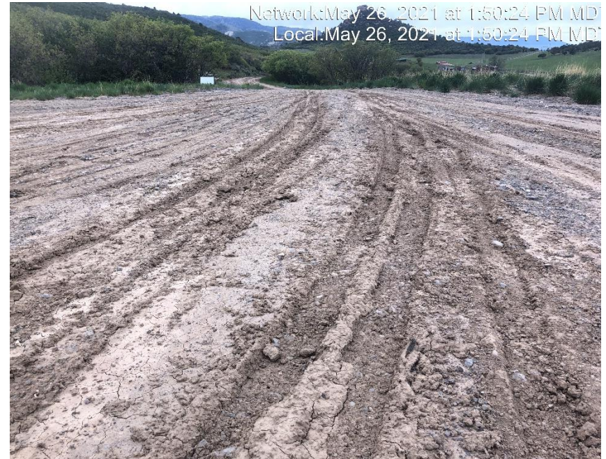
Photo #3946 No form of tracking BMP at entrance to location.
