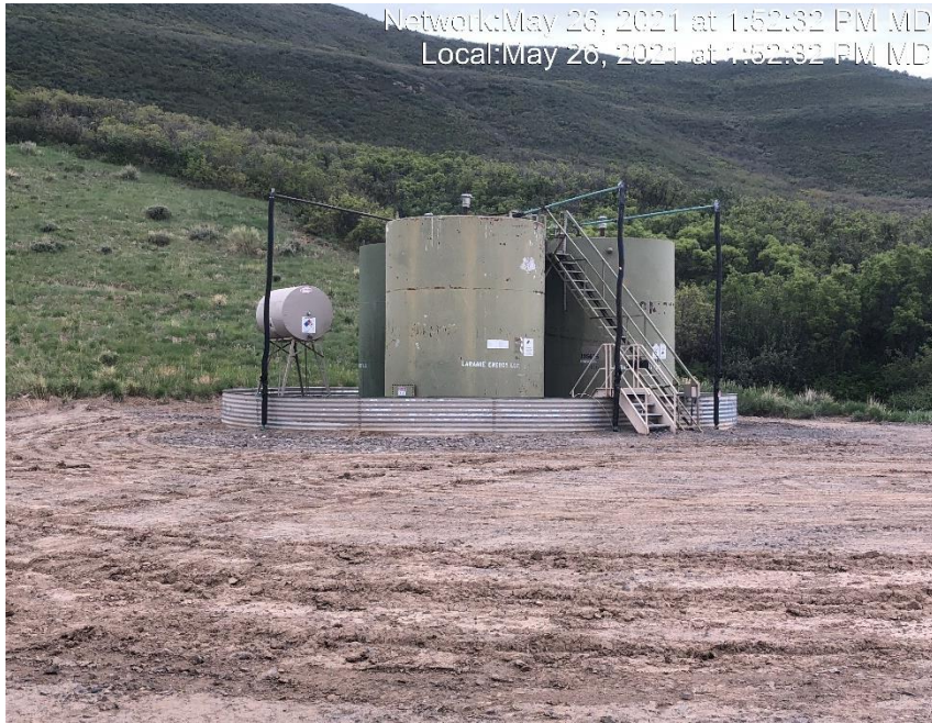
Photo #3947 No battery sign located at the tank battery.
