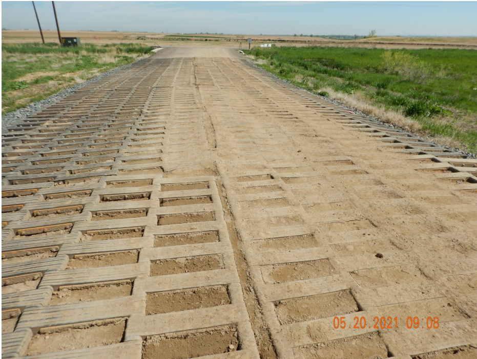
Photo 6. Photo taken from the entrance of location, facing North. Photo illustrates the vehicle tracking device BMP is in need of maintenance.
