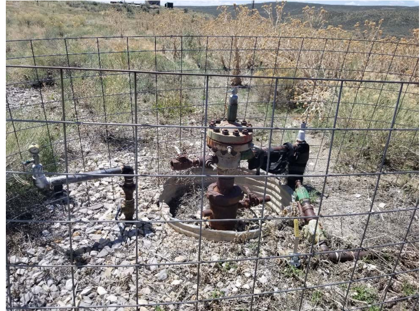
Photo 2. No bradenhead access apparent.
