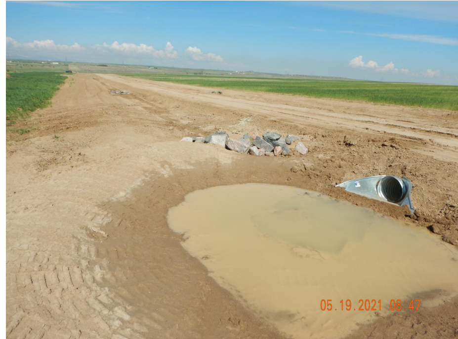
Photo 10. Photo taken from the entrance of the facility, facing West. Photo illustrates no outlet protection has been installed.
