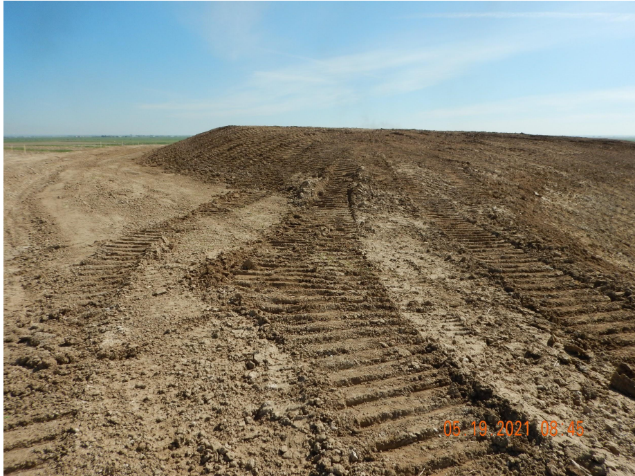
Photo 7. Photo taken from the northwestern location, facing North. Photo illustrates the topsoil stockpile which has been temporarily stabilized with equipment tracking.
