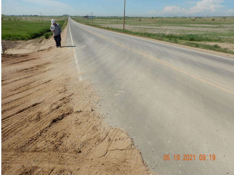
Photo 2. Photo taken from the entrance of location, facing South. Photo illustrates no vehicle track out was observed.
