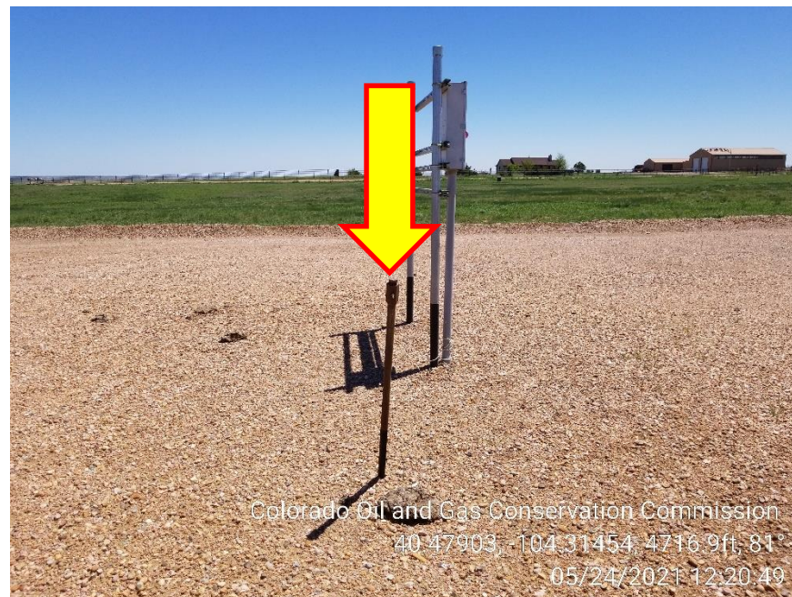
Photo 2 – Unmarked Riser south of Wellhead
