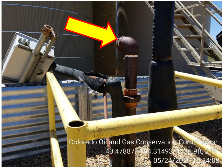
Photo 11 – Unmarked Riser at Tanks
