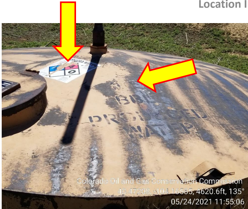
Photo 5 – NFA and Capacity Level have faded; no longer visible
