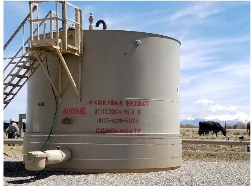
Photo 4. Tank label inaccurate.
