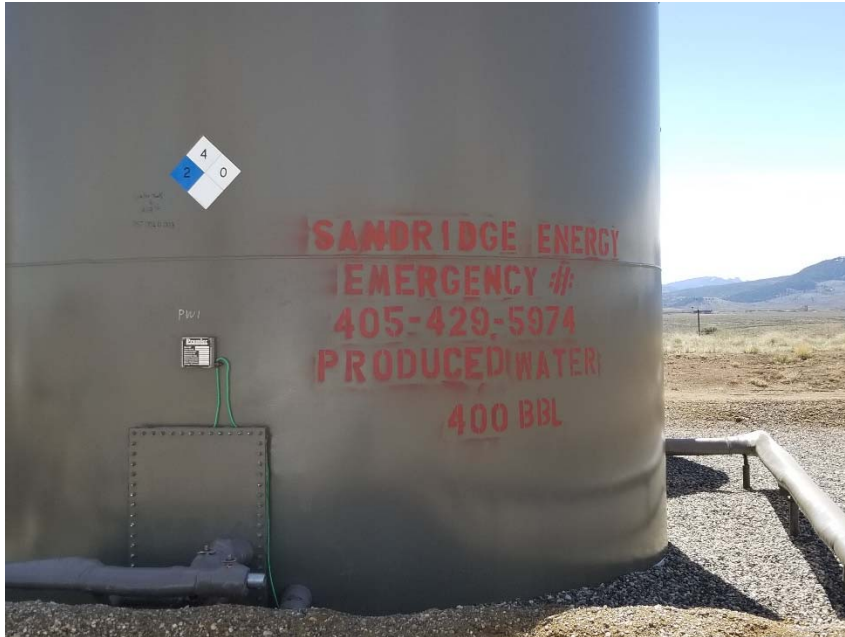
Photo 4. Tank label incomplete/inaccurate.
